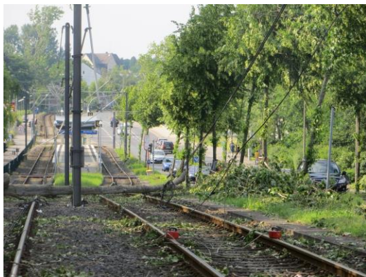
Fig. 3.2. Damage to suburban rail system. Photo: Rainer Klute.
