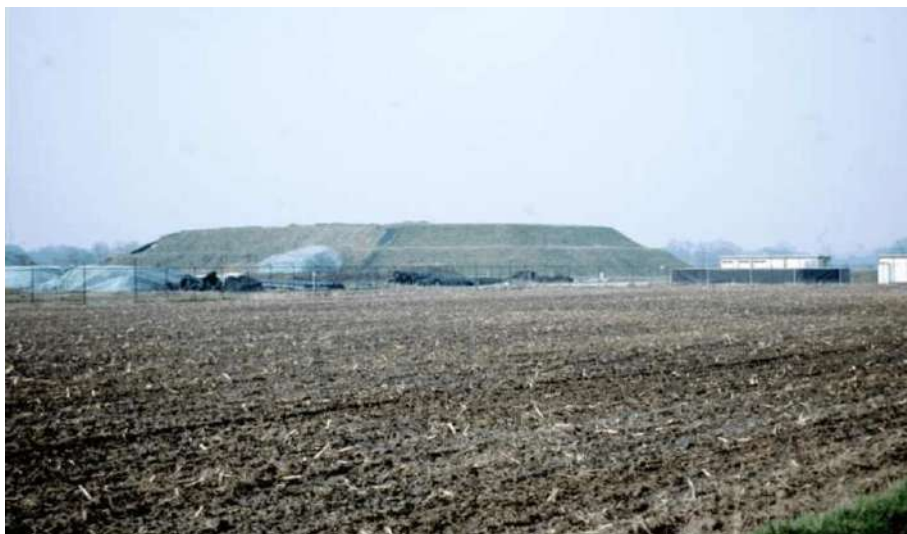
Photo 2. Temporary storage of 200,000 tonnes of contaminated soil
