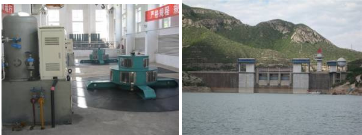
Plate 6 Power generation station Upstream FID at second reservoir
