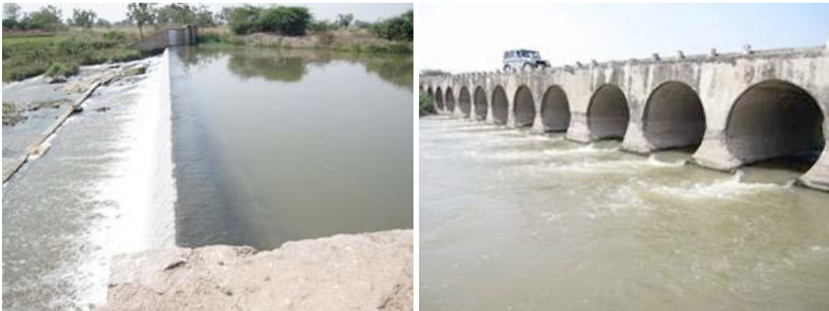
Plate 10 Downstream of Shahapur BC, weir with possibility of monitoring the flow (left) - bridge which should be equipped with measurement device (right)
