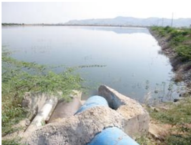
Plate 4. Shahapur City Domestic water Reservoir fed by irrigation pipe.
