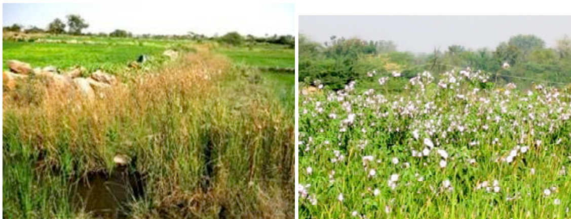
Plate 7 Drainage services: invasion of vegetation
