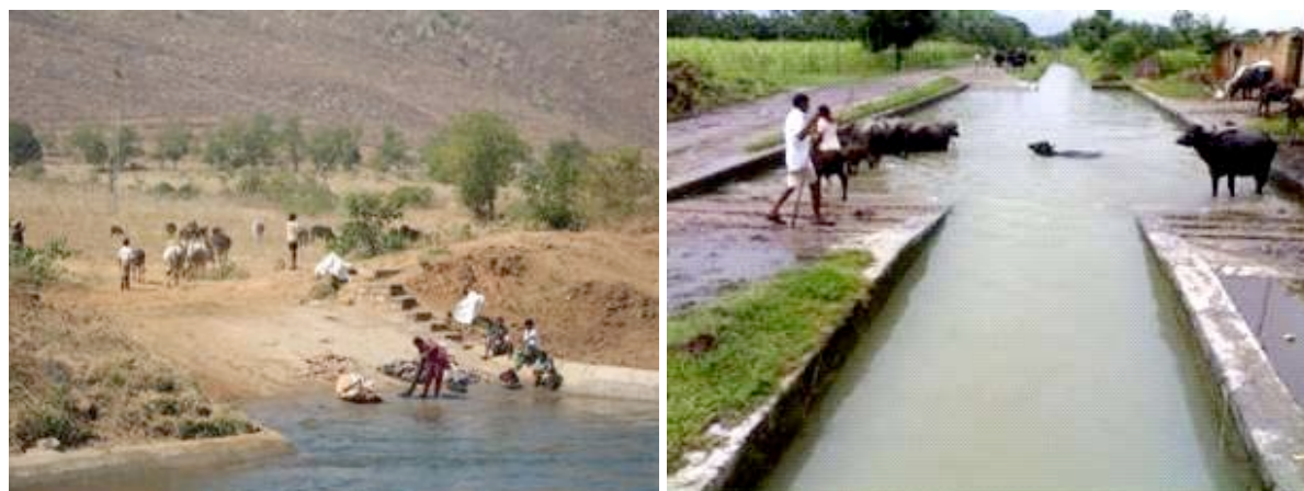
Plate 16 Examples of ramp easing water access for animals (Bhadra Karnataka-left; Main Ganga UP -right) .
