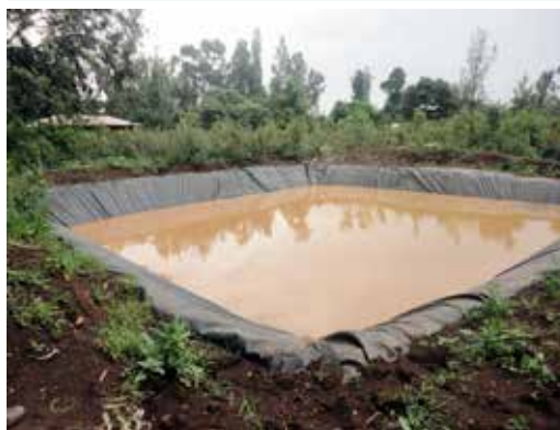
Figure 3: Rainwater harvesting pond, with geo-membrane lining to reduce seepage loss
