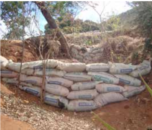
Figure 1: A reclaimed gully using sand gunny bags in Kibao watershed
