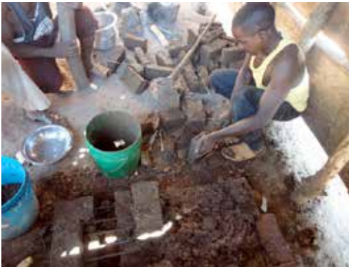
Figure 3: Preparing the basement for the improved stove
