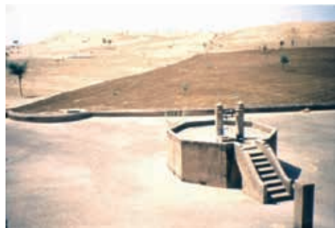
Figure 9. A tanka or tanki (also called a kund in some places). This image is of a 250-year old kund in Churu District, Rajasthan. It is for harvesting rainwater in a region where the groundwater is saline
