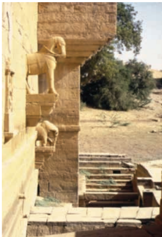
Figure 1. The water level in Amarsagar pond, Rajasthan, was built in the fifteenth century. The water level is measured by the statues of elephants and horses
