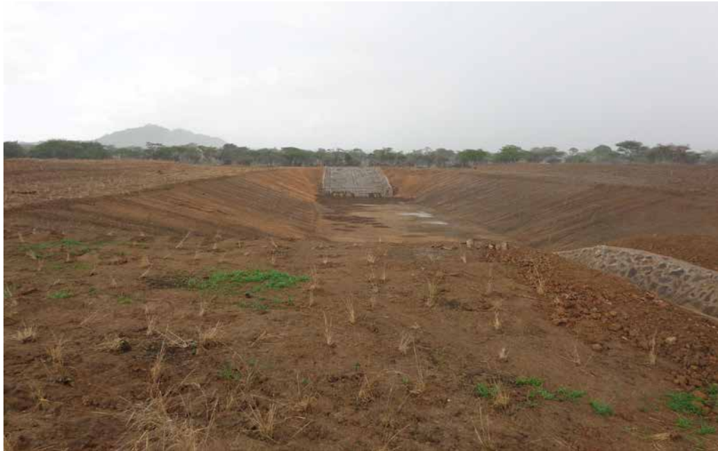
Figure 4: Excavated valley tank
