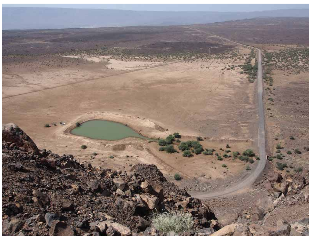
Figure 2: Example of an embankment pond fed by a road culvert
