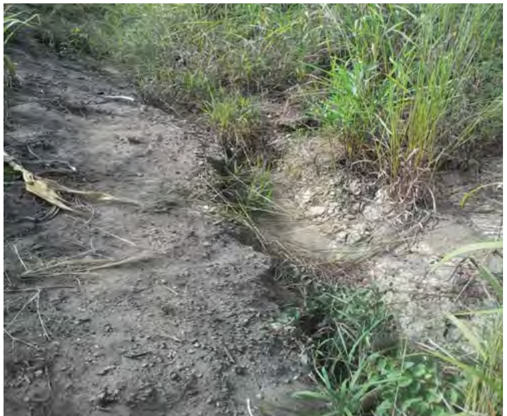
Sheet and rill erosion Kanduku
