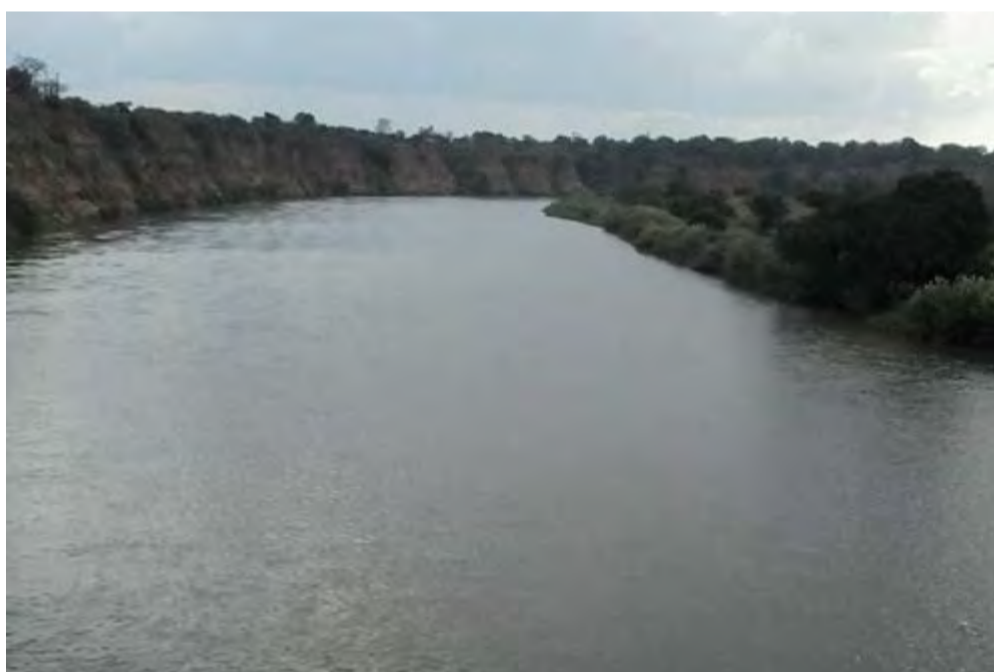
Riverbank erosion at Shire River (near Kamuzu bridge)
