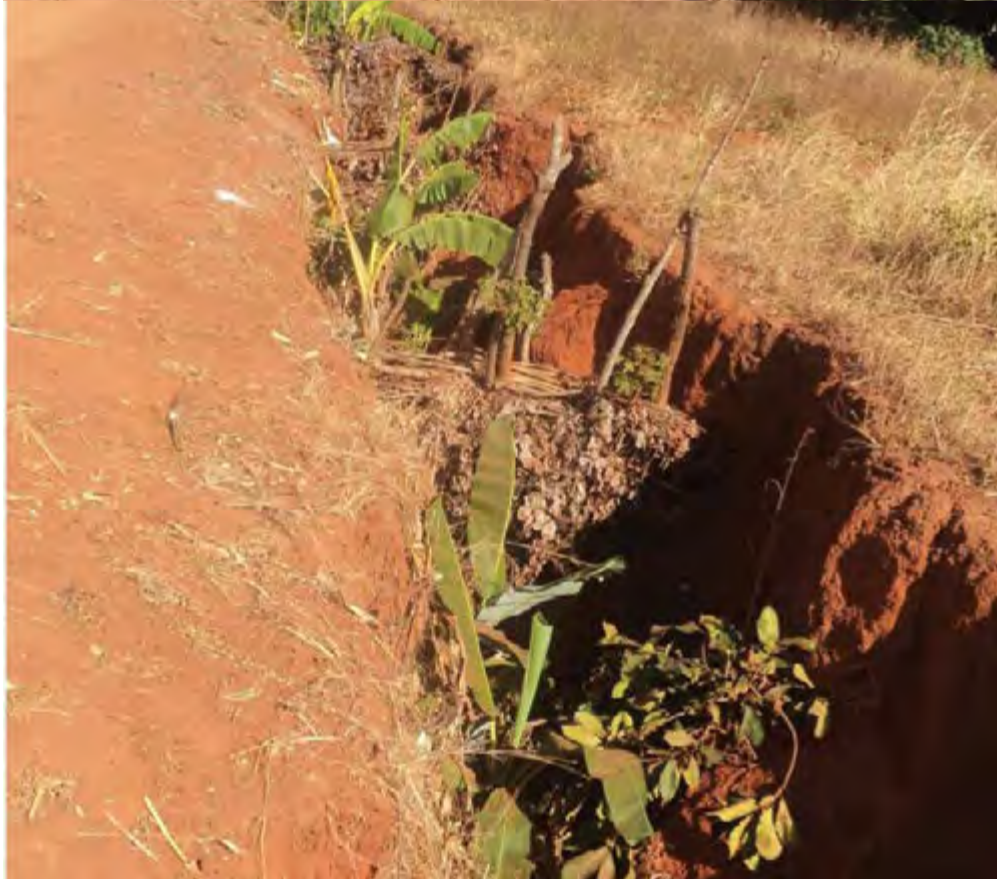
Gully erosion control at Chikweya Village by Chisikwa conservation group
