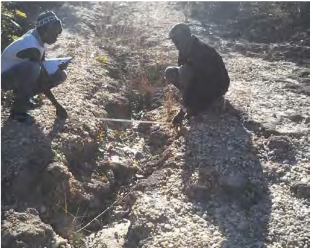
Rill erosion at Joel Shawa
