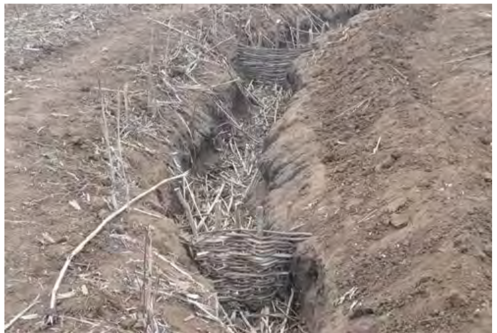
Rill erosion control at Mbepula
