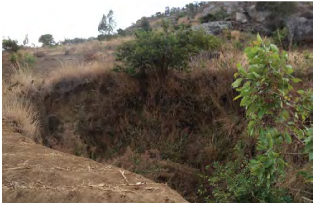
Gully erosion at Zidana village
