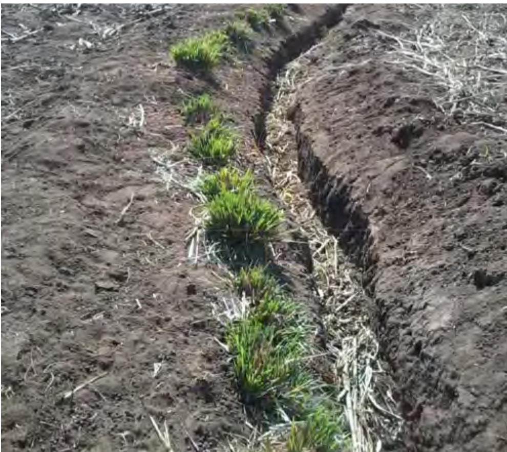
Cut-off drain at Khembo at Magoti EPA
