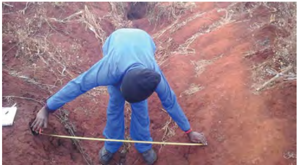
Sheet and rill erosion at Thondo in Chikwatula EPA
