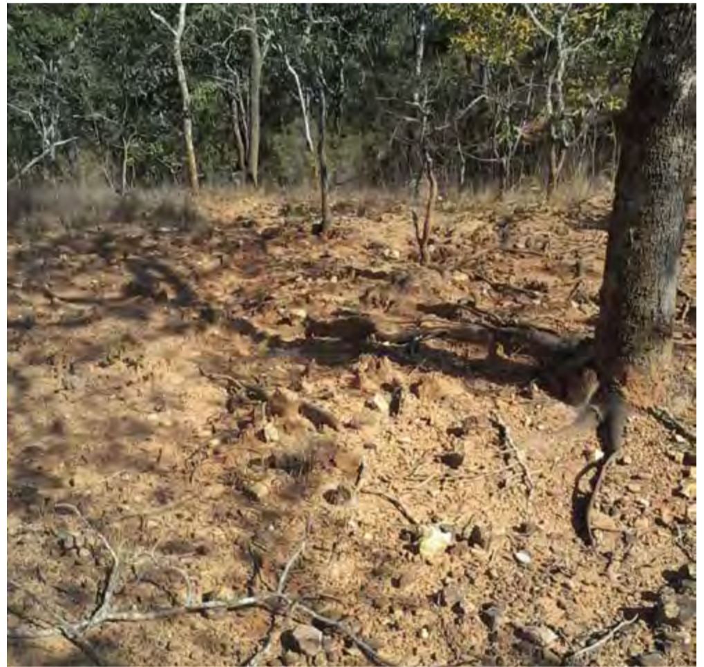
Sheet erosion at Sanga Topsoil loss rate
