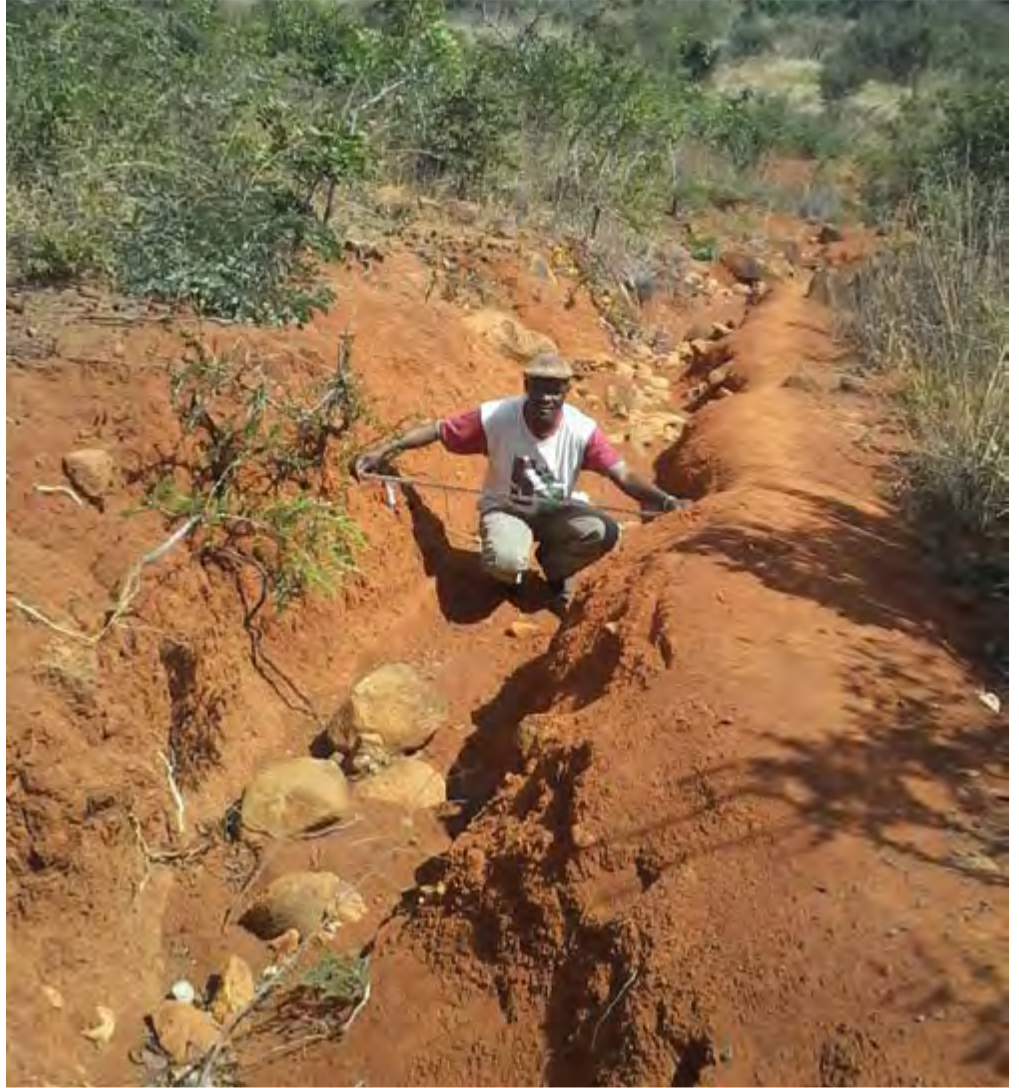
Rill erosion at Katula
