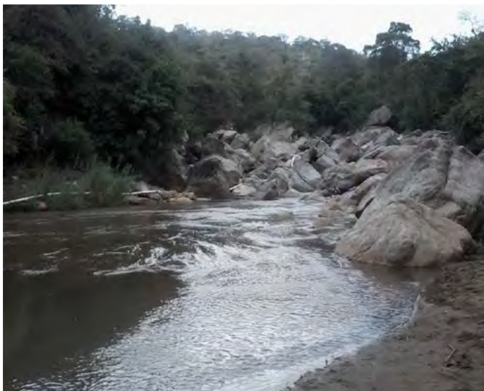
Maintenance of cover on riverbanks at Maperera
