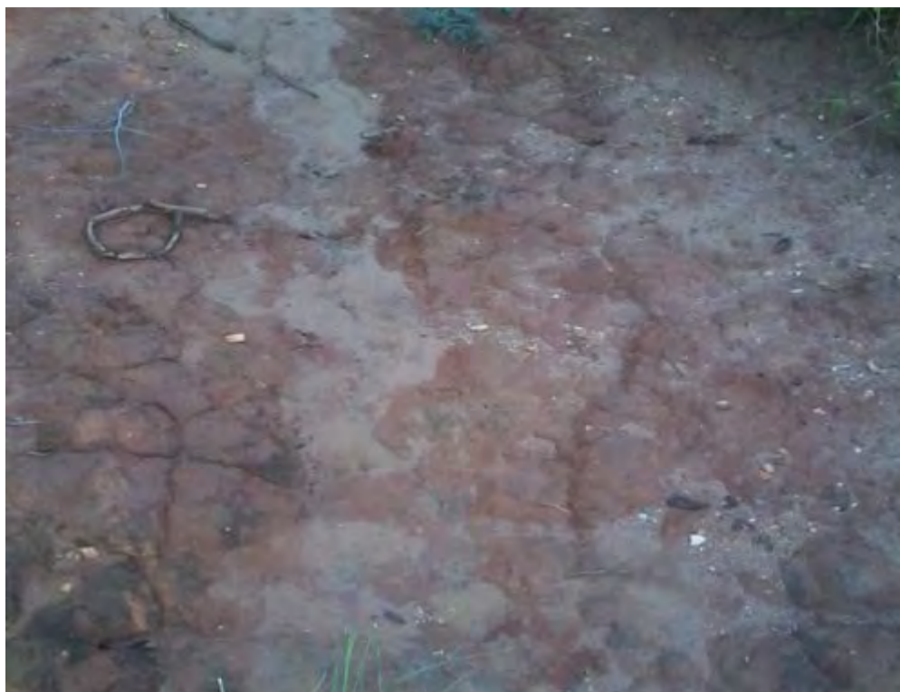
Sheet erosion and soil surface hard-setting at Katunga
