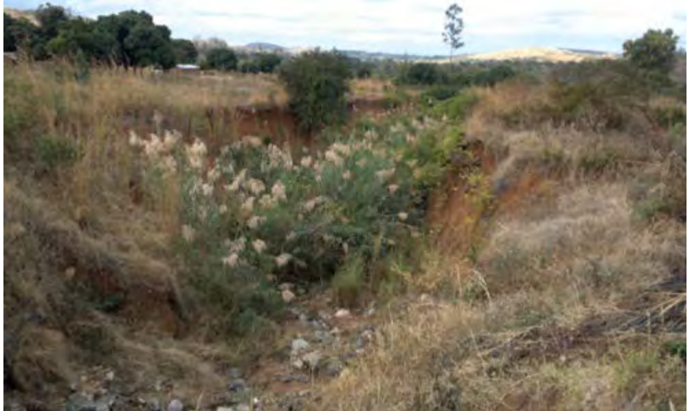
Gully erosion at Nauma
