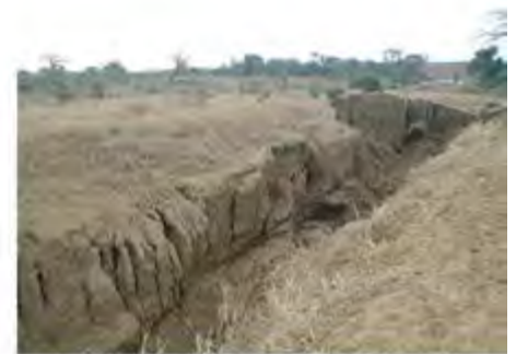
Rill and gully erosion
