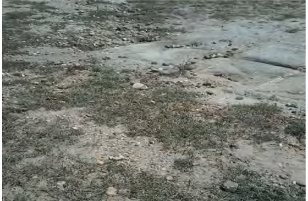
Sheet and gully erosion at Nkundika
