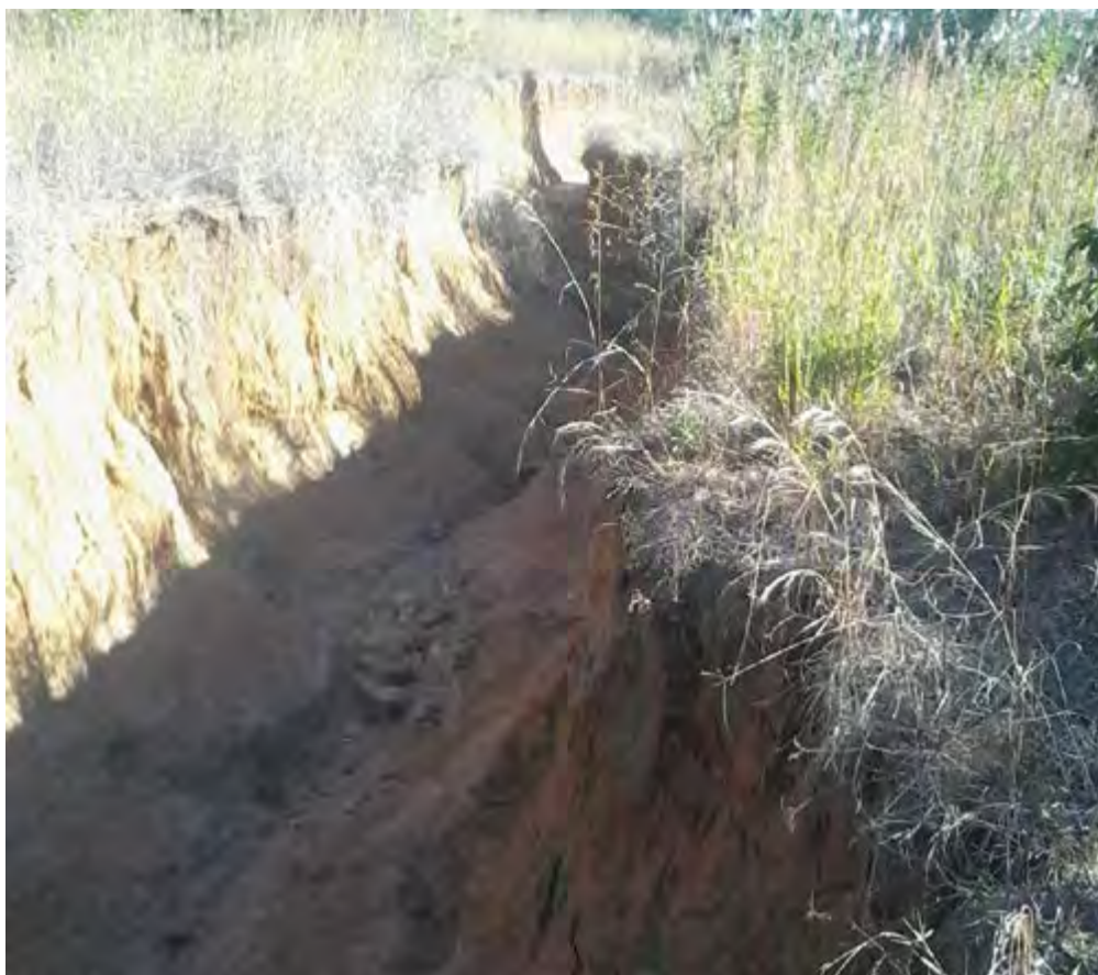
Gully erosion at Chilipula
