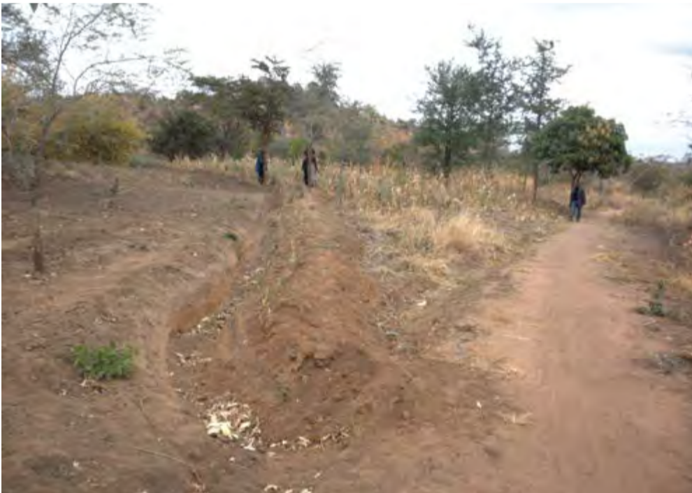
Cut-off drain at Khembo at Magoti EPA
