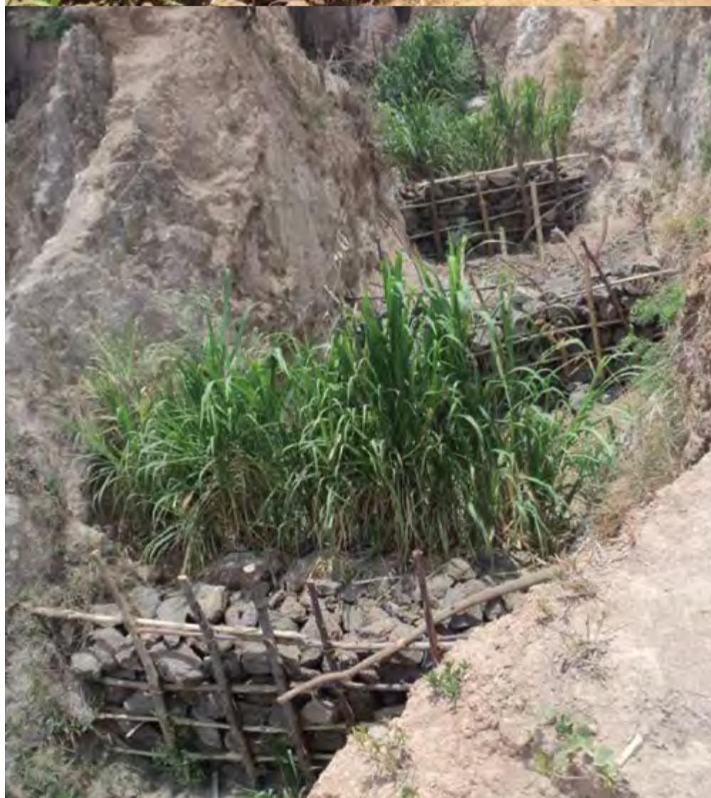
Protection of gully floor and gully erosion advancement
