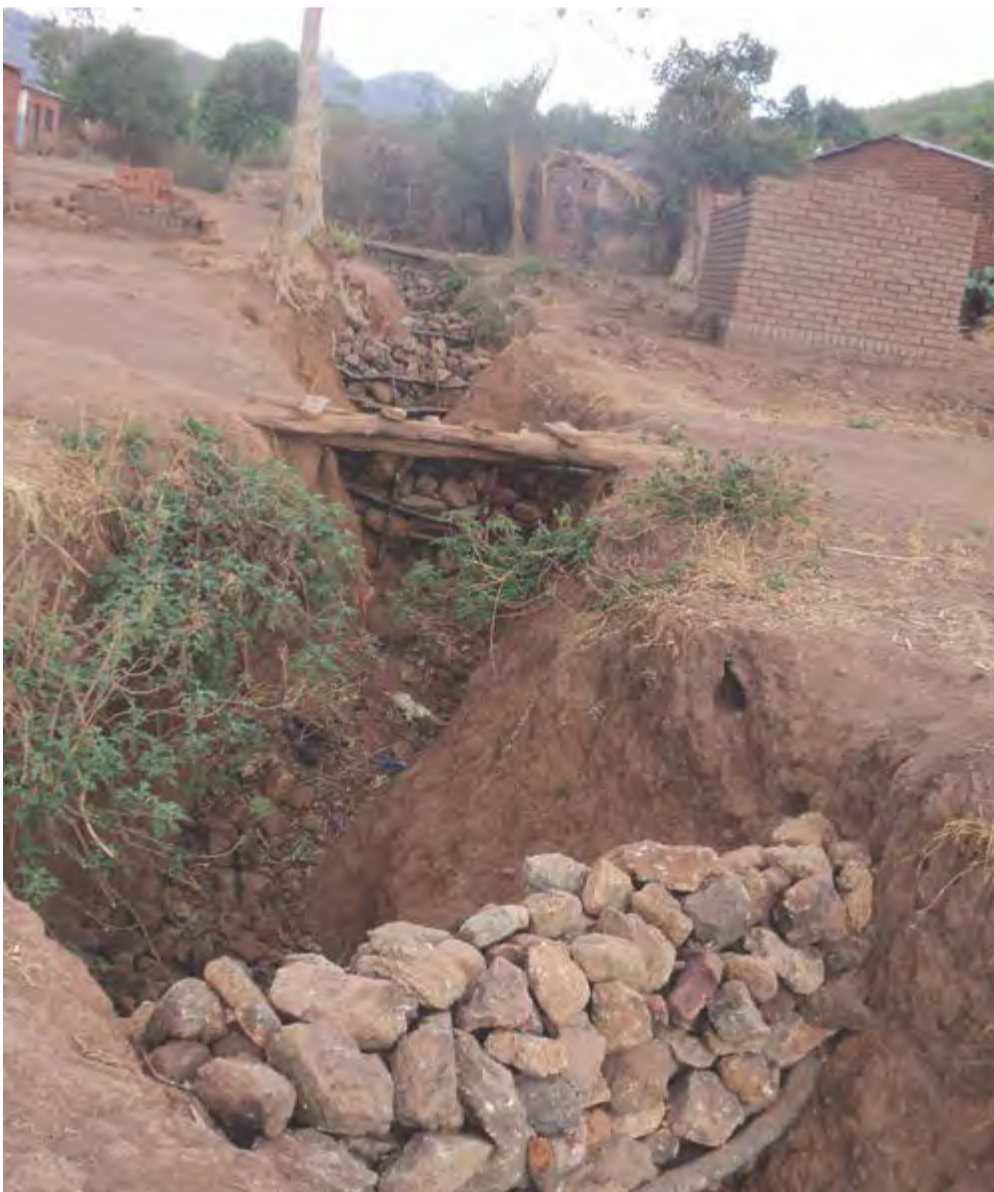
Gully erosion control at Chilobwe
