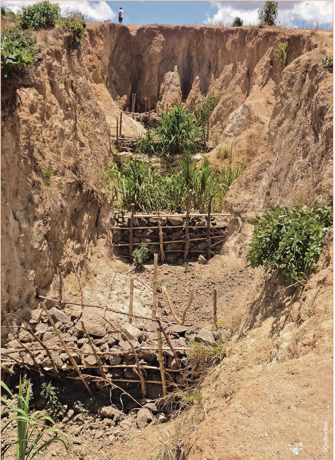
Figure 3: Sediment trapping using stones and growing vegetation, Dedza, Malawi.
