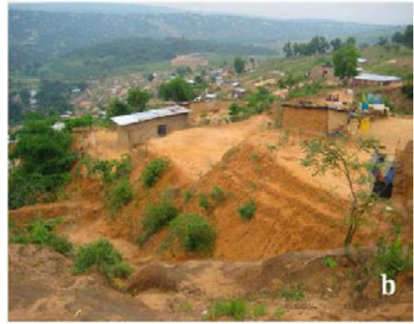
Figure 2: Ravine appeared following the completion of a collector (a) Terraced urban development on an erosion-sensitive site (b)
