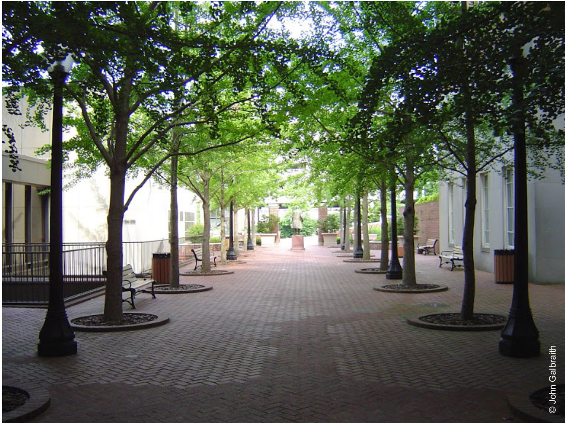
Photo 35. Trees surrounded by pervious brick pavement
