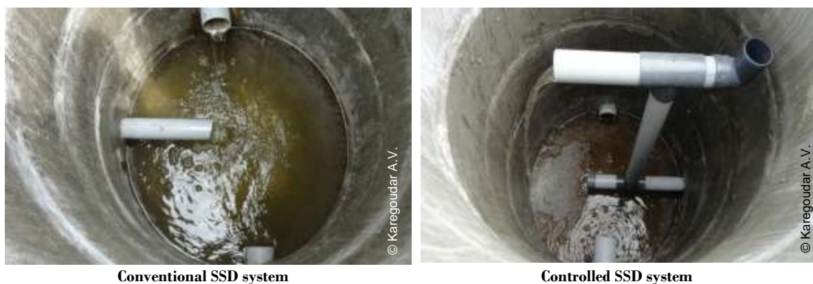
Figure 1. Conventional & Controlled SSD systems
