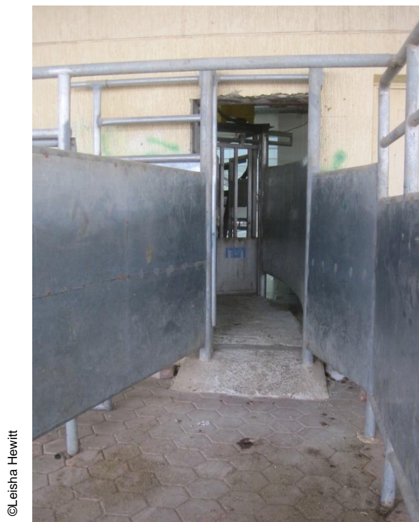
Figure 7. Cattle handling facility with single-file race leading up to restraint
