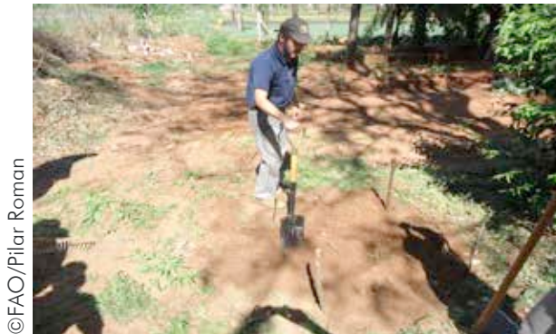
Figure 46 Cleaning the pile area
