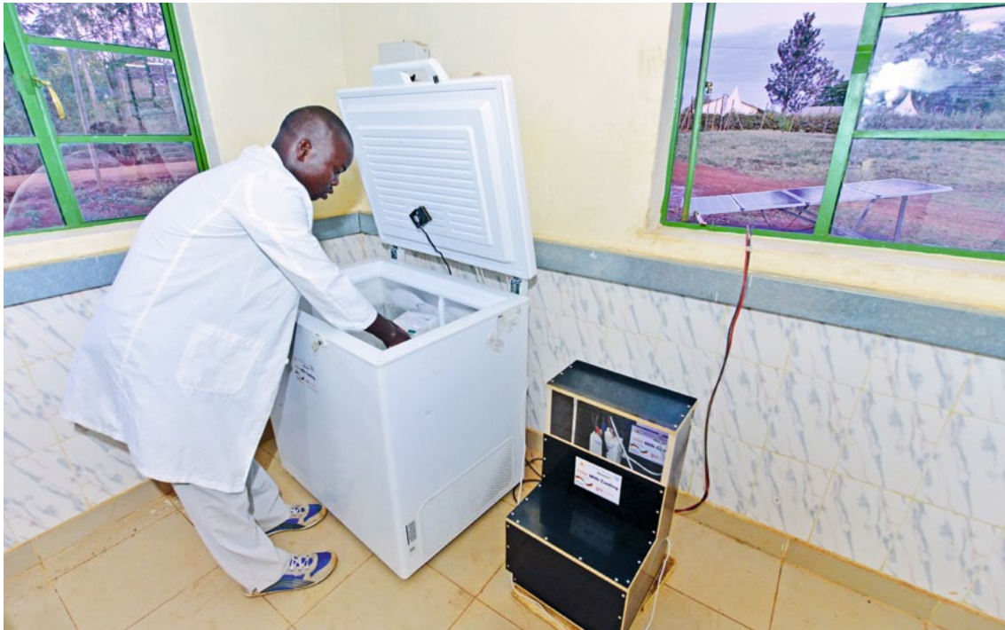
When possible, the use of batteries should be avoided in solar cooling systems. The systems developed by the University Hohenheim/Germany for example uses ice as thermal storage. Source: © GIZ/Alex Kamweru
