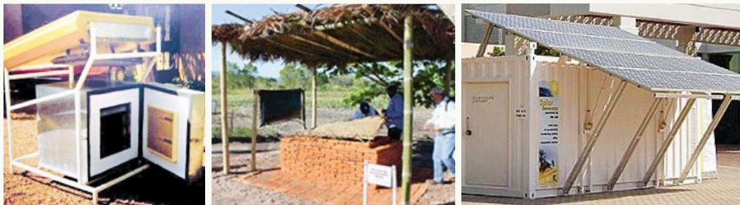
FIGURE 4.29. Examples of a passive chiller, solar thermal refrigerator and solar PV-powered cold storage room.
