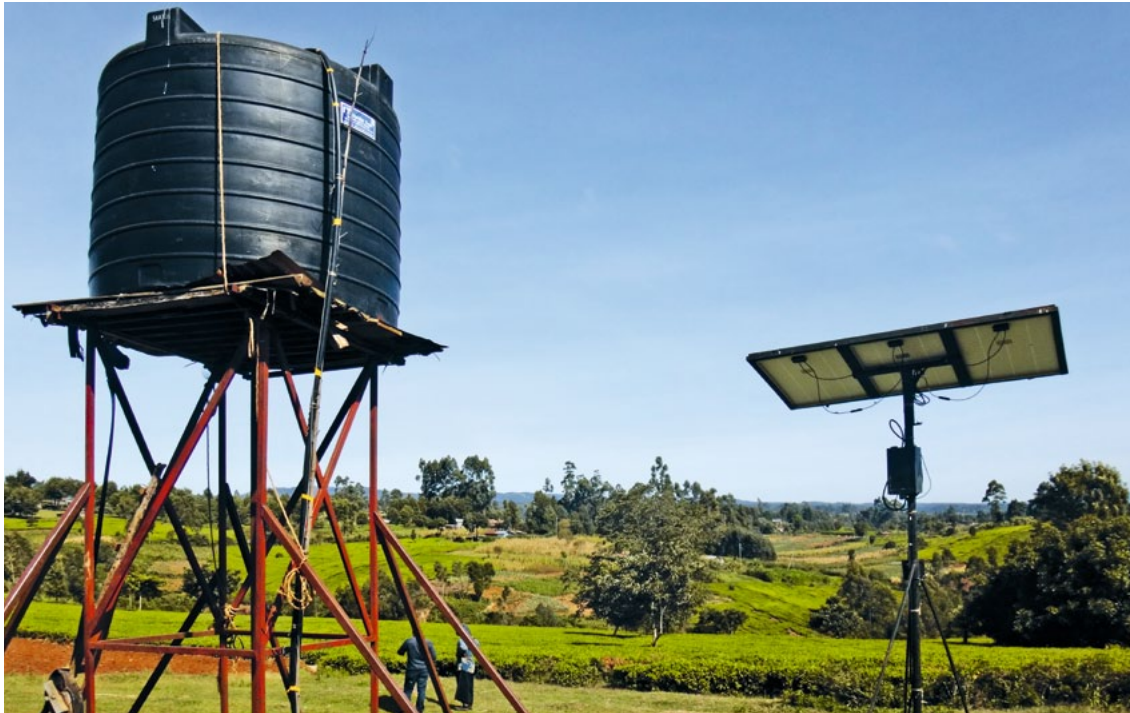
In remote rural areas grid electricity is often not available and fossil fuels are costly. Solar irrigation systems allow for coping with such circumstances. Source: © GIZ/Fehrenbach
