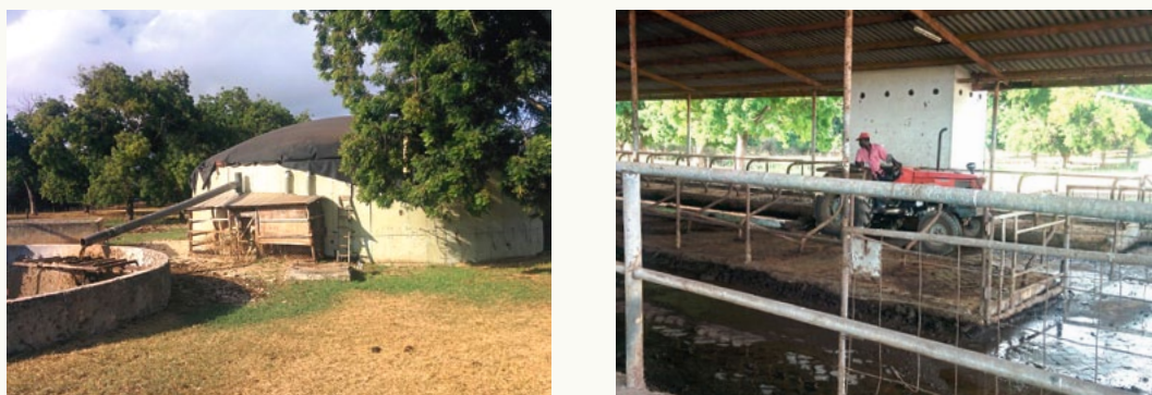
FIGURE 4.4. Biogas plant in Kilifi, Kenya: effluent storage tank, digester and shed containing the gas engine and generating plant.
