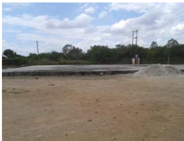
Concrete sun-drying platform outside the warehouse
