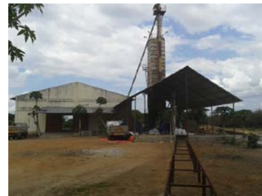
Rails from the warehouse to the dryer next to the factory
