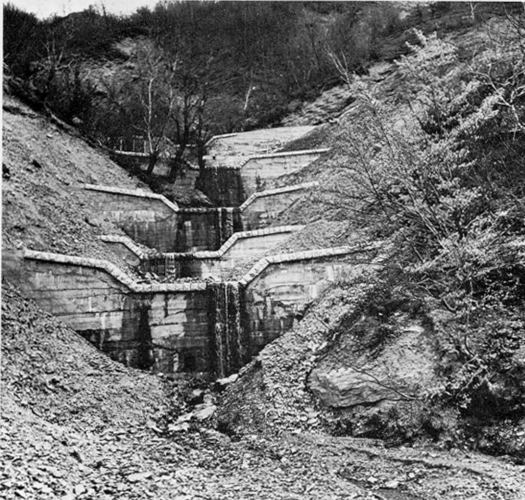
FIGURE 58. - Permanent structures controlling a gully. (Yugoslavia: FAO Photo.)
