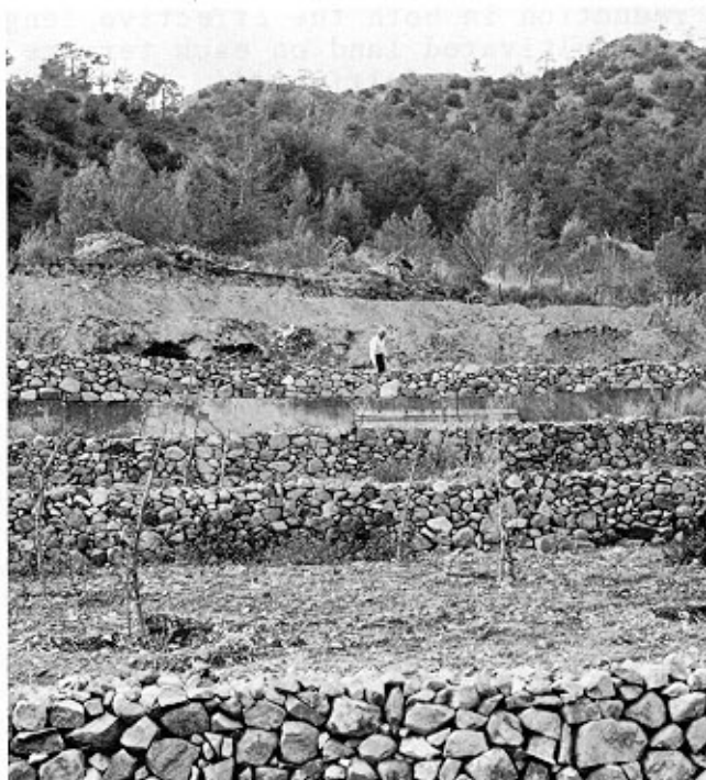
FIGURE 49. - Staggered bench terraces on a hillside overlooking flooded valley bottom in Nepal. (FAO Photo by R. Vroom)
