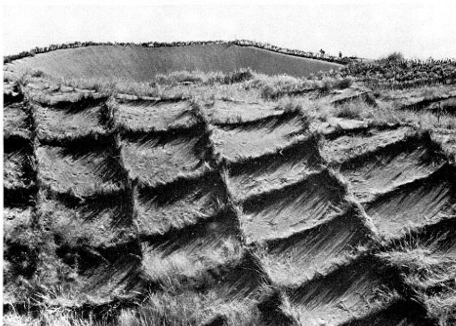
FIGURE 62. - Stabilization of sand dunes. (Chile: FAO photo by H. Hull)
