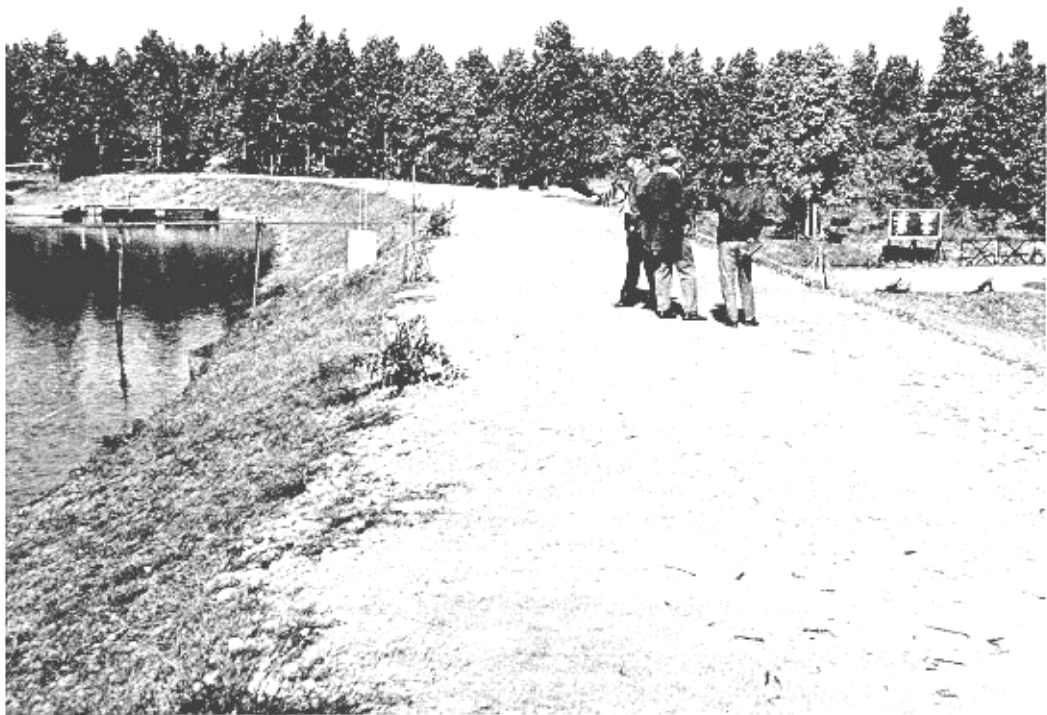
Fig. 20 Good vegetation restores the eroded landscape owing to better soil and moisture conditions created by sediment detention tanks - Damodar Valley Corporation, eastern red soil region
