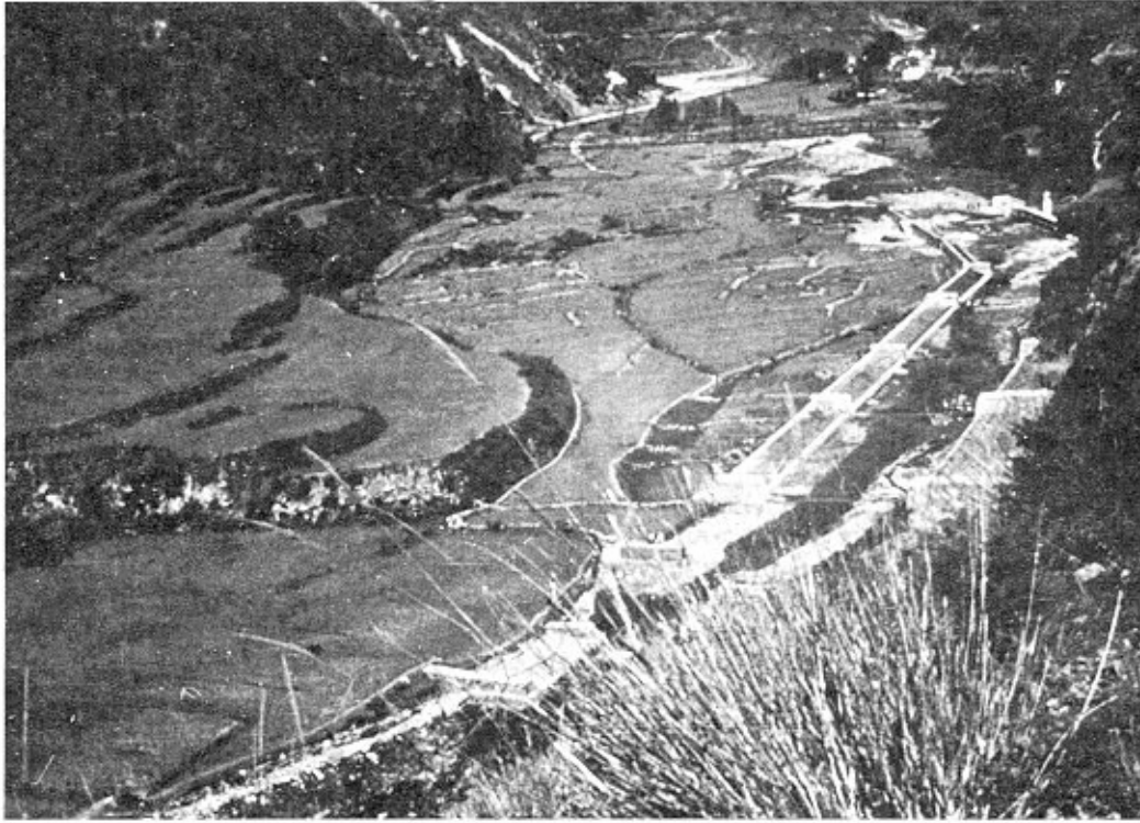
Fig. 13 Torrent control by rivetments, with shell structures supplemented by contour planting of Salix in the Ramganga catchment of the northern Himalayan region.
