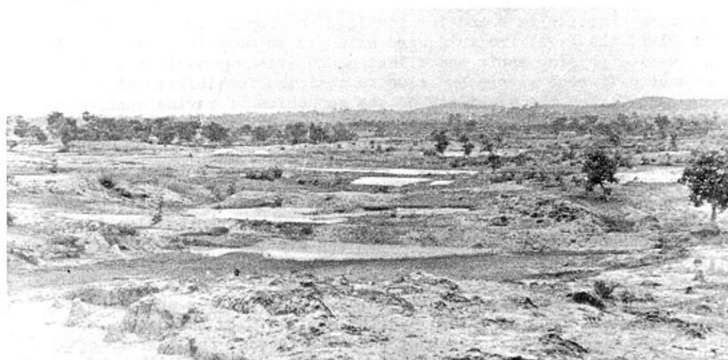
Fig. 12 Controlling erosion and restoring gullied lands by creating small ponds and developing paddy benches in the Mayurakshi catchment in the eastern red soil region
