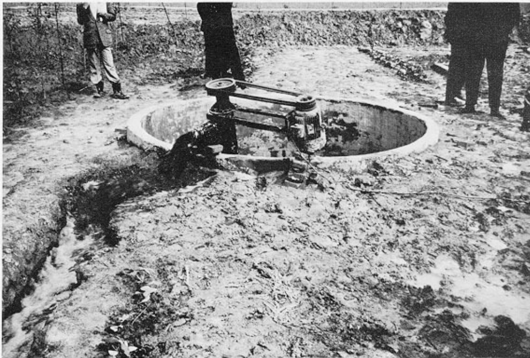
Fig. 46 Outlet of large size bio-gas plant. Effluent pumped into irrigation drain. Cheng Hsiang Production Brigade, Jiangsu Province.
