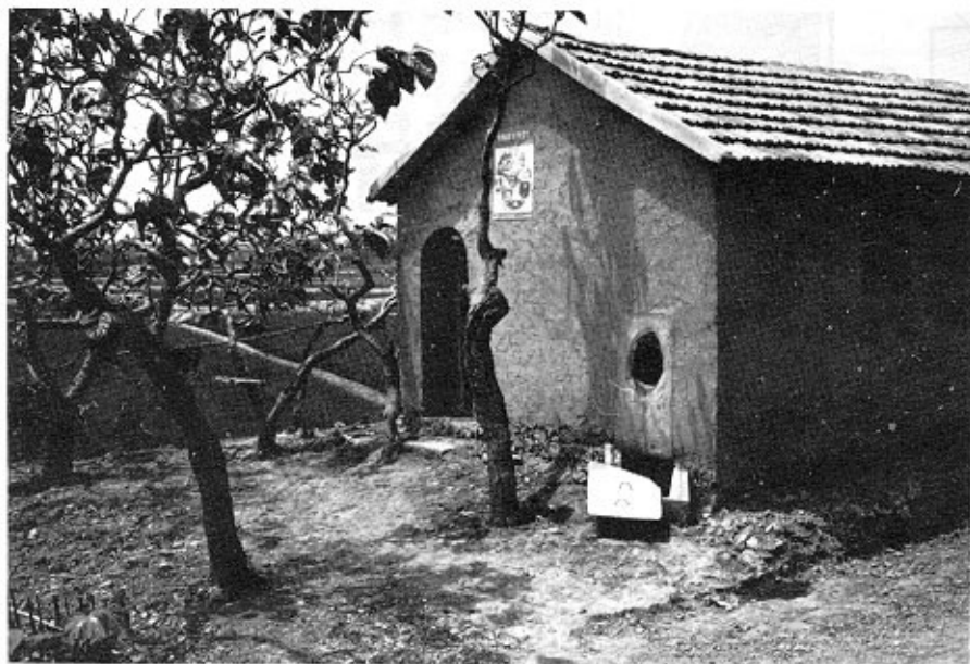
Plate 19. Outside the pigsty of Plate 18, showing an inlet in the wall for adding household waste to the biogas unit and, at ground level, the biogas unit outlet.
