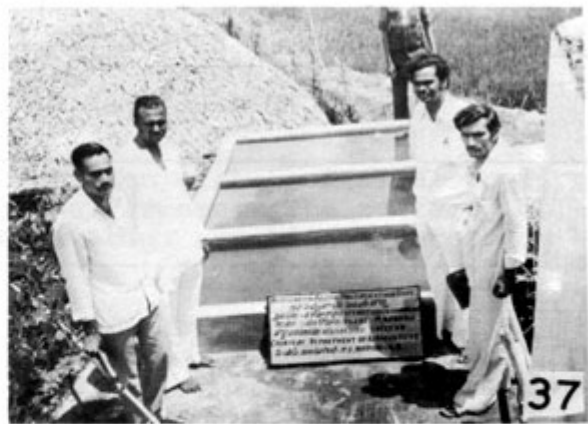
Figure 37 Farmer's algal production unit built on the roof-top of his house
