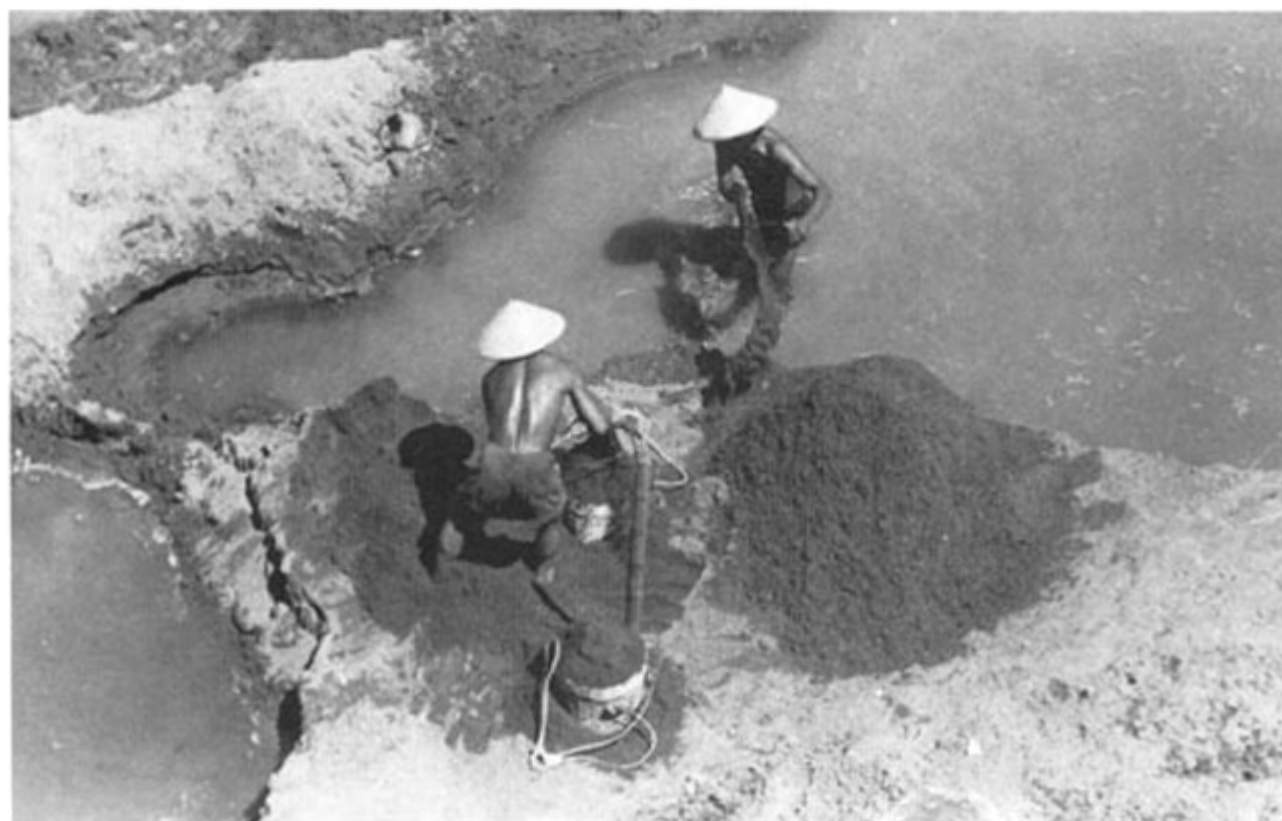
Fig. 28 Workers removing silt from Solo River in Java, Indonesia. Silt was deposited in the river due to erosion on uplands (FAO photo)
