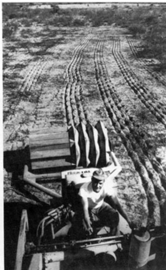
Fig. 106 Land imprinter (photo provided by R.M. Dixon (USDA-ARS))
