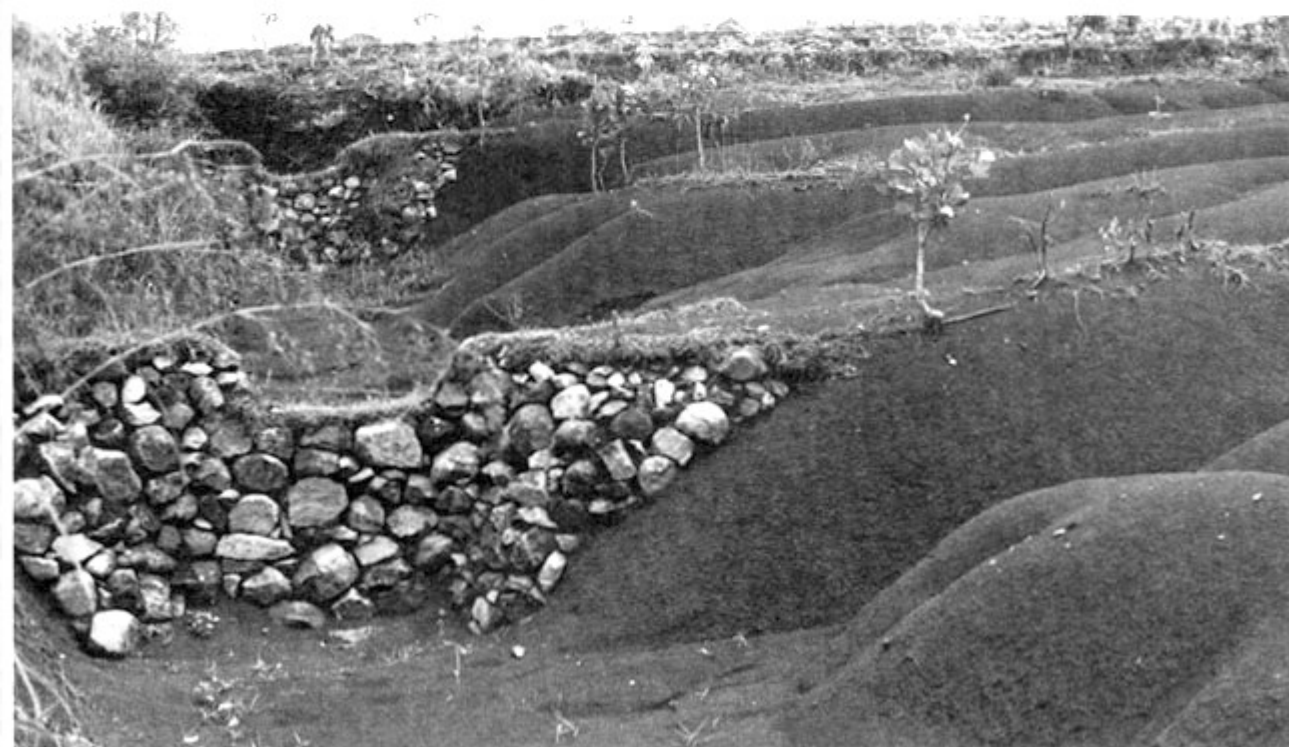
Fig. 100 Check dams in gully. Silt settles behind the dams, thus filling the gully, enabling terrace construction and rehabilitation of a critically eroded area in the Upper Solo Valley, Indonesia (WFP photo, issued by FAO)
