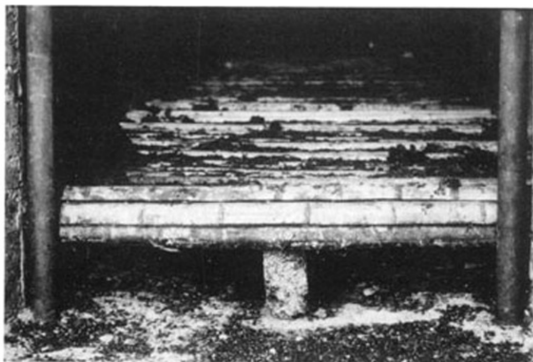
Plate 19 Details of bamboo floor of coffee pulp composting pit. Narrow gaps between the bamboo poles allow the pulp to drain and air to enter underneath the composting mass Source: FAO filmstrip Uses of Coffee Pulp
