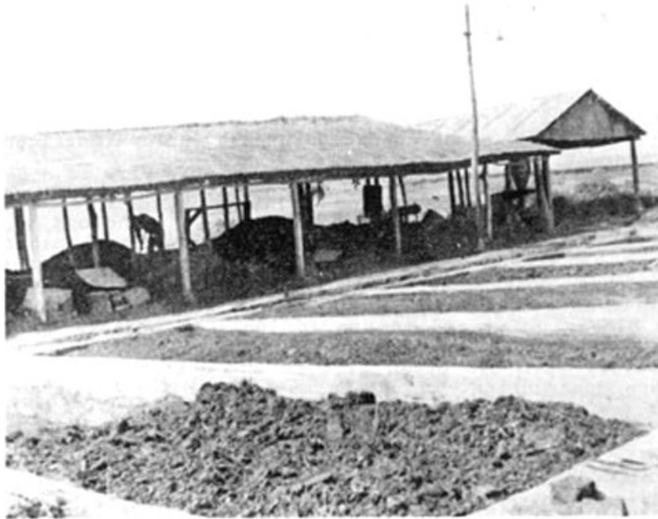
Plate 20 Pits constructed above ground for refuse-night soil composting. Hammer mill for crushing and sieving facilities under cover at rear Source: Gotaas (1956) and van Vuren (1949)
