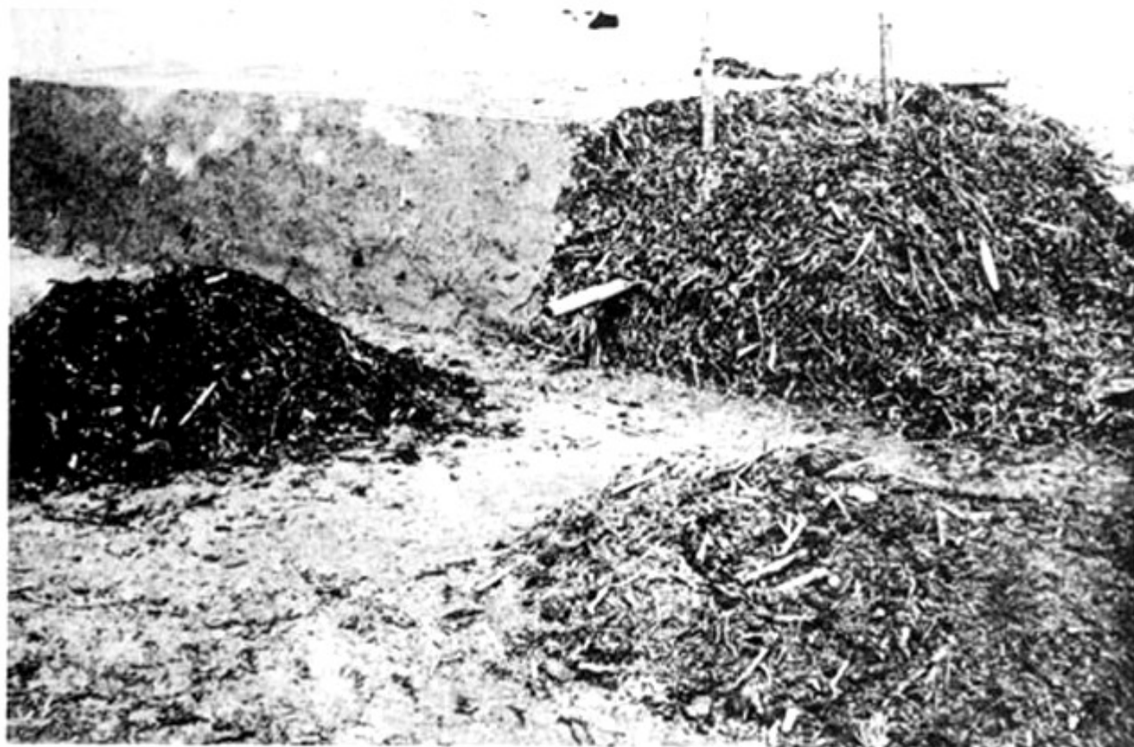
Plate 16 Chinese high temperature heap, construction details showing bamboo poles in place to form aeration passages Source: FAO (1978c)
