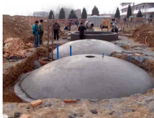
FIGURE 6.7 Bio-organic reactors at household scale
