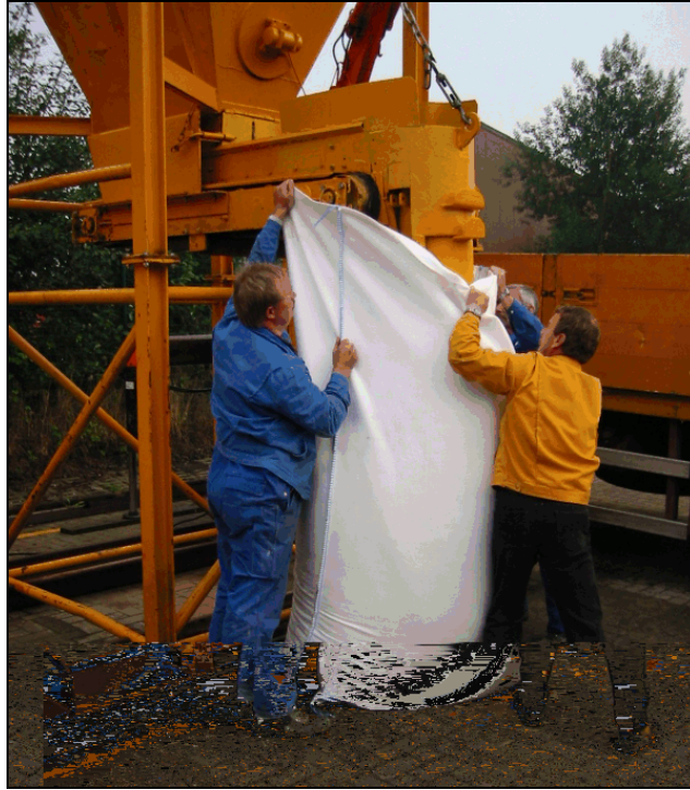
Figure 5.5. Filling 1.0 metric tonne geotextile container with sand. (photo from NCHRP Project 24-07(2), courtesy Colcrete – Von Essen Inc.)
