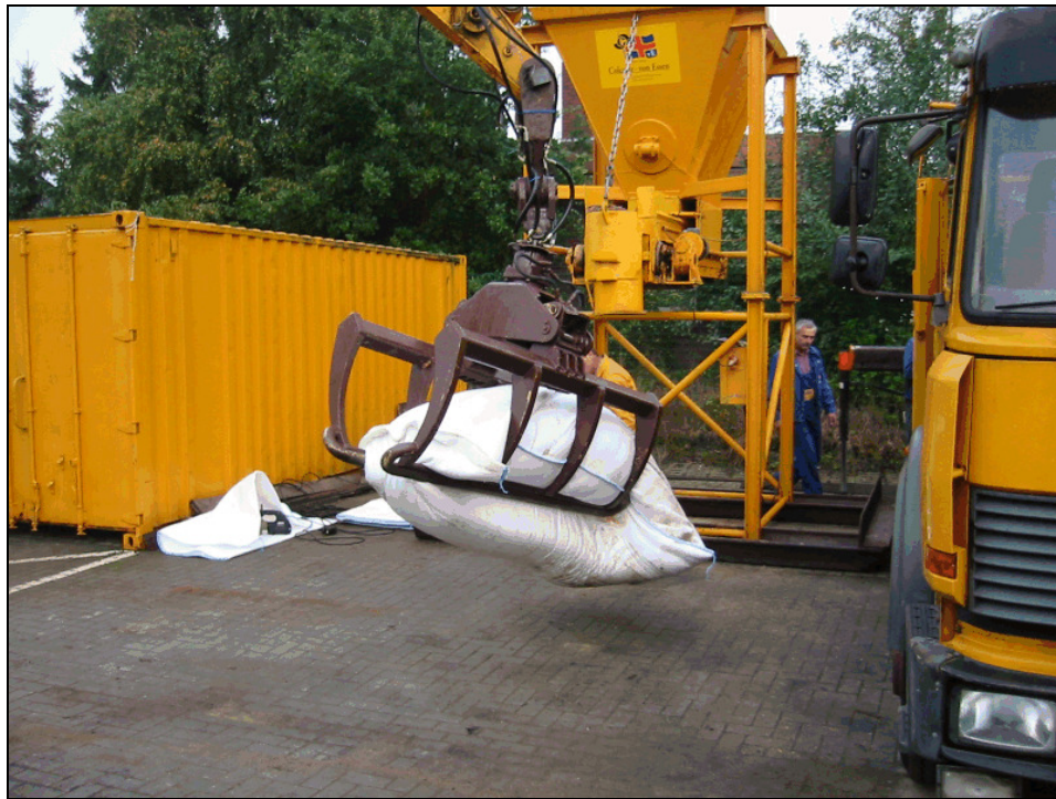
Figure 5.6. Handling a 1.0 metric tonne sand-filled geotextile container. (photo from NCHRP Project 24-07(2), courtesy Colcrete – Von Essen Inc.)
