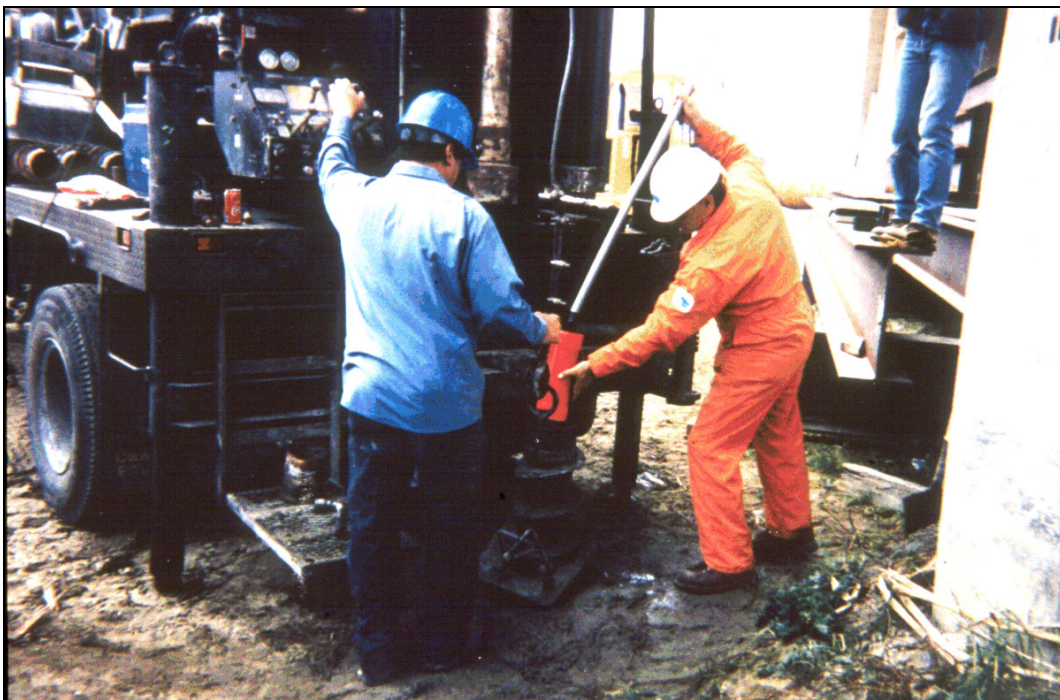
Figure 9.30. Installation of float out device on Salinas River Bridge near Soledad, CA.
