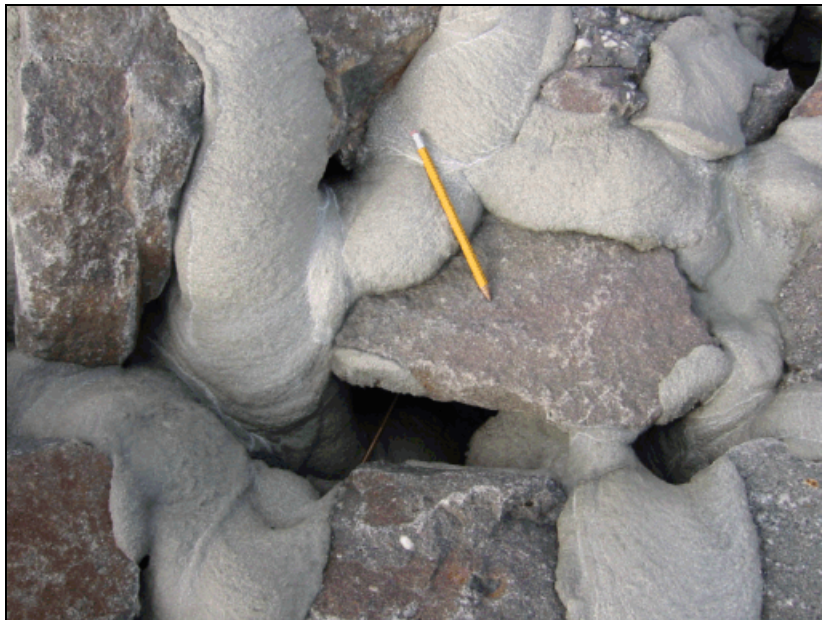
Figure 12.1. Close-up view of partially grouted riprap.
