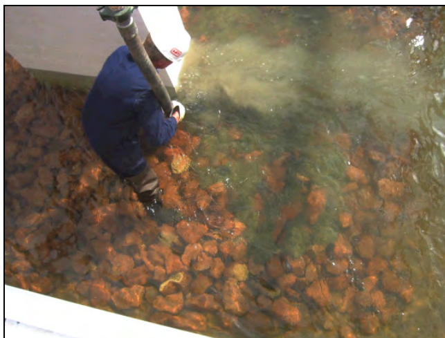
Figure 12.11. Underwater partial grouting of riprap.
