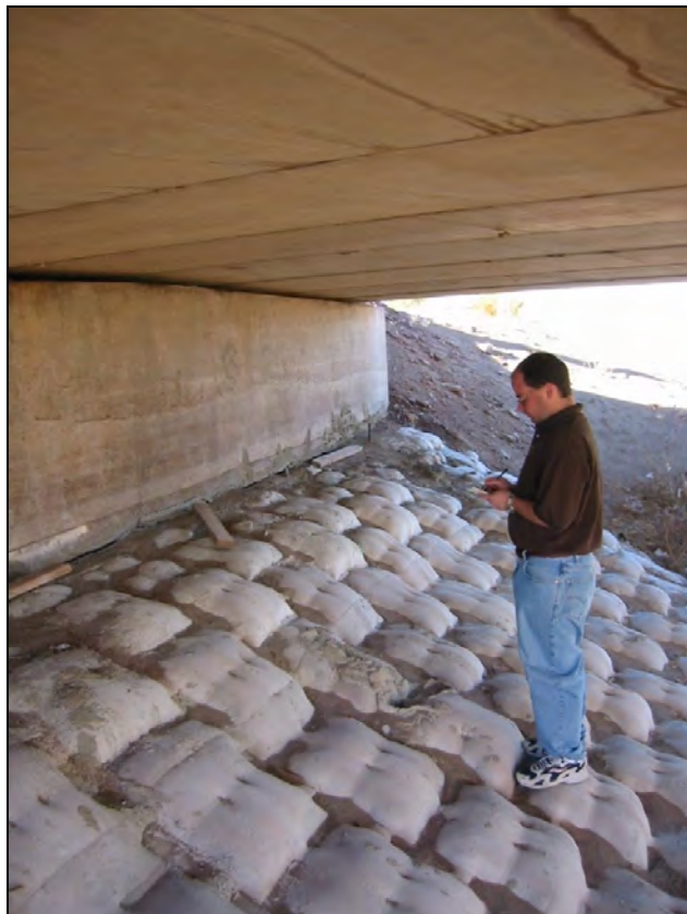
Figure 9.2. Grout-filled mat used for scour protection at a bridge abutment.
