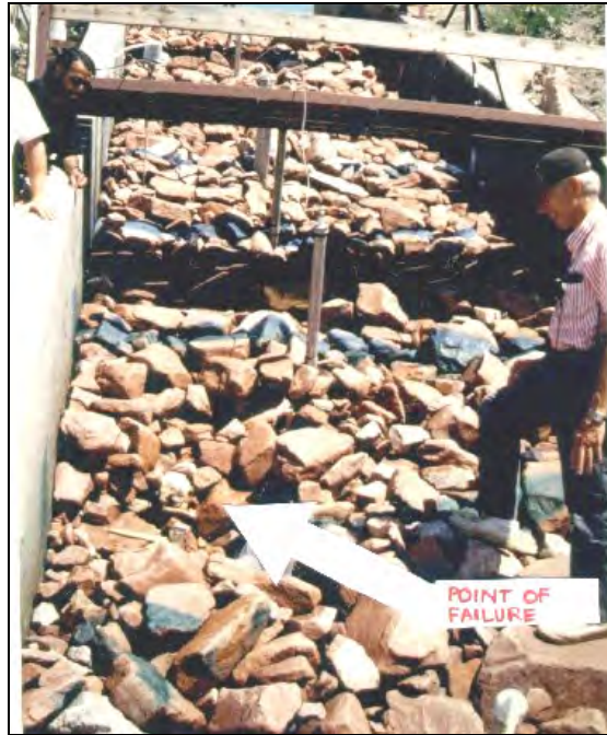
Figure 5.7. Riprap failure in 1994 tests ( d_{50} = 1.27 ft (386 mm))
