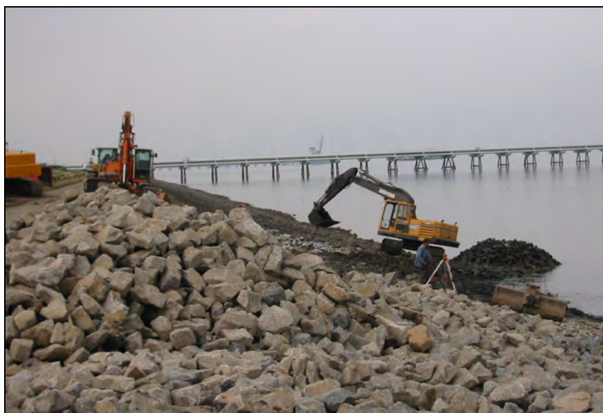
Figure 4.11. Placing riprap with hydraulic excavators.
