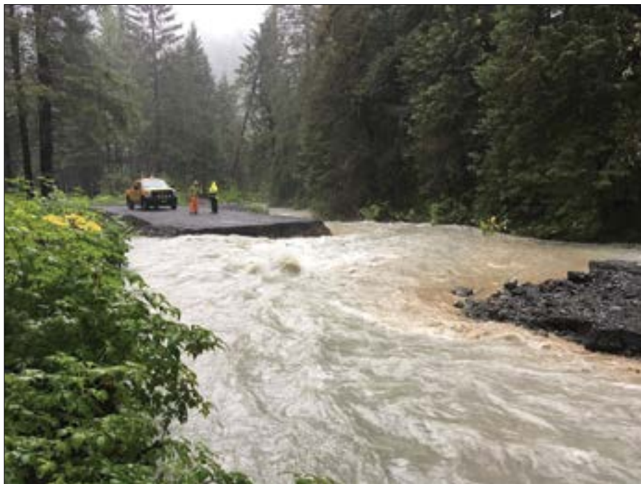
Figure 3.7—Roads that wash out repeatedly, as shown here in Chugach National Forest, are good candidates for decommissioning. (Photo by USDA Forest Service)
