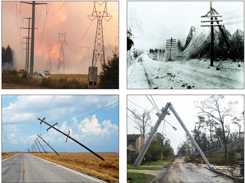
Figure 5: Examples of Weather-Related Electrical Grid Disturbances
