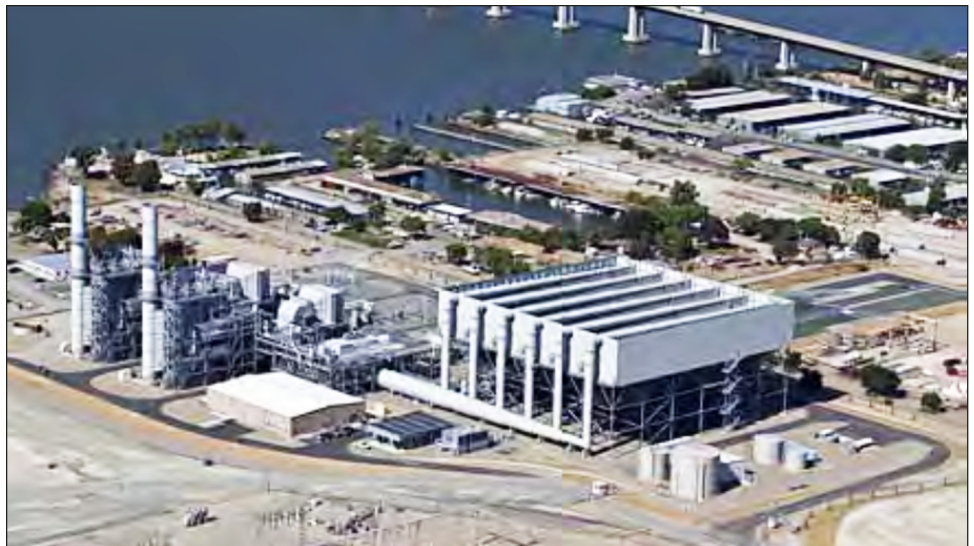
Figure 11: Gateway Generating Station
