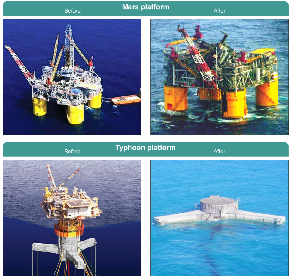
Figure 3: Damage to Mars and Typhoon Platforms from Hurricanes Katrina and Rita, 2005
