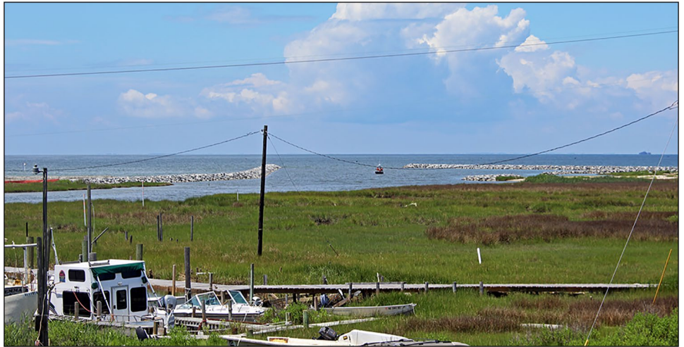
Figure 4: Completed Rhodes Point Jetty, Smith Island
