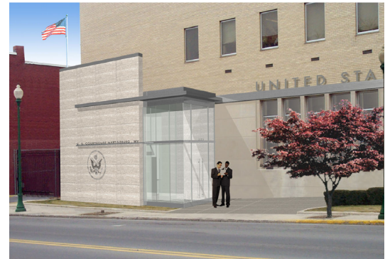
Figure 7.24 The new security pavilion is designed to integrate with the overall character of the building, utilizing a similar material palette and picking up existing architectural design cues. It creates a more welcoming and clearly defined approach on King Street.
