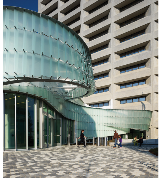
Figure 7.17 The new lobby extension provides a sharp contrast with the original building, clearly articulating the main entrance. The warm tones of the frosted glass and the natural forms project a welcoming image to visitors.
