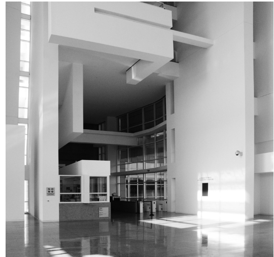
Figure 7.38 The security station in the lobby is designed with geometry and materials that match the architectural language of the space, allowing it to virtually "disappear" instead of competing with the lobby's architectural character.
