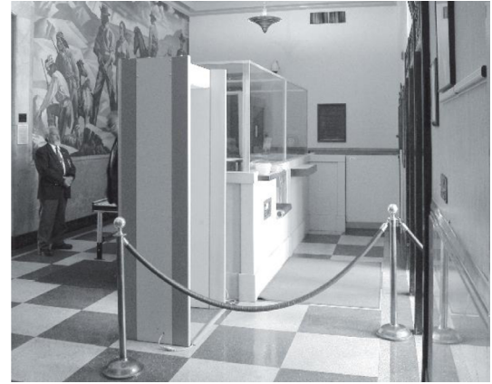
Figure 7.48 The redesigned security station uses ballistic glazing on all sides to preserve views of the mural.
