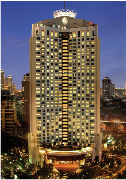
INTERCONTINENTAL, JAKARTA. JMBM assisted the owner of this landmark Jakarta hotel in terminating a long-term, no-cut, management agreement with a top luxury brand, selecting a new operator and rebranding the hotel as the InterContinental Midplaza.
