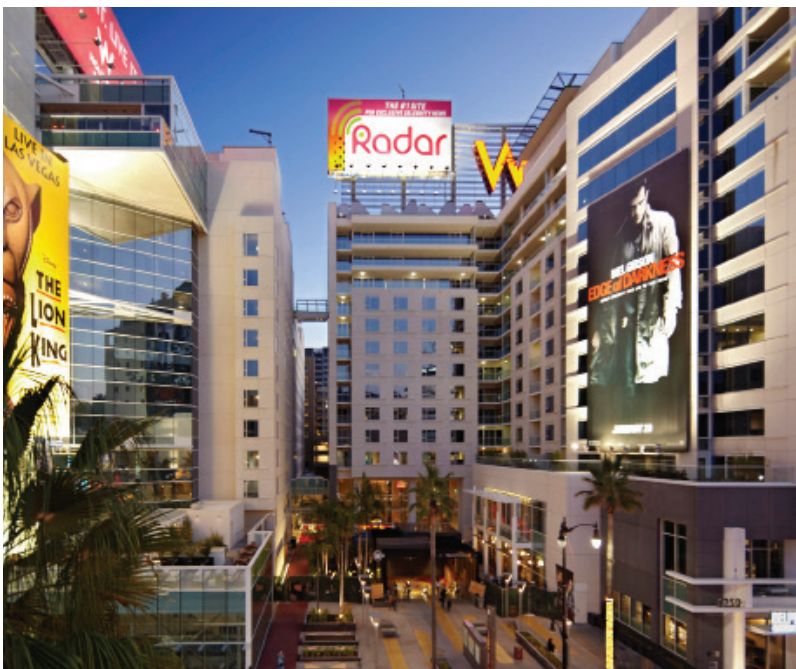
W HOTEL, HOLLYWOOD. We worked on many aspects of this mixed-use hotel property, including land use, almost $300 million of senior debt and mezzanine financing for development, and EB-5 financing for the Drai's Vegas-style night club and the Delphine fine-dining restaurant at the hotel.
