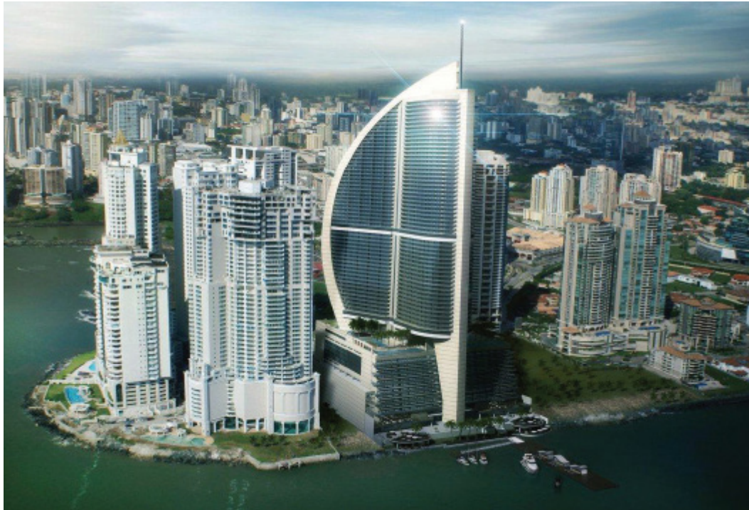
TRUMP OCEAN CLUB INTERNATIONAL HOTEL & TOWER, PANAMA CITY. Luxury hotels like this often provide the spark plug to energize and create value with high-end mixed-use for hotel-anchored residential, condo hotel, retail and office projects. We have represented the Trump Organization and other clients on more than 100 hotel mixed-use projects throughout the U.S., Latin America, the Caribbean, Asia and Europe.
