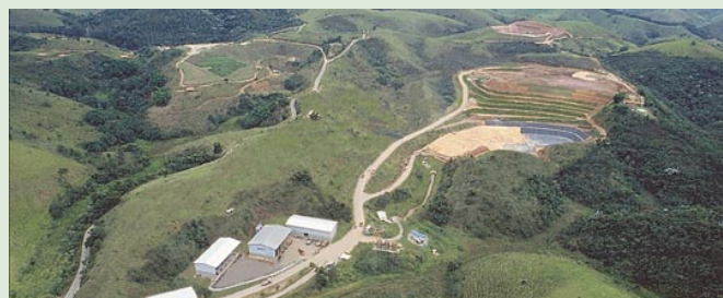
Figure 10.10: ONYX SASA Landfill Gas Recovery Project .VES landfill, Trémembé, Sao Paulo State
