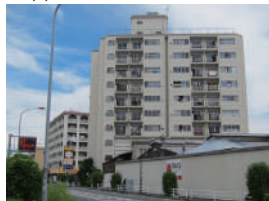
<Outer appearance before construction>
