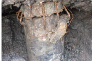
<Damaged pilings>
