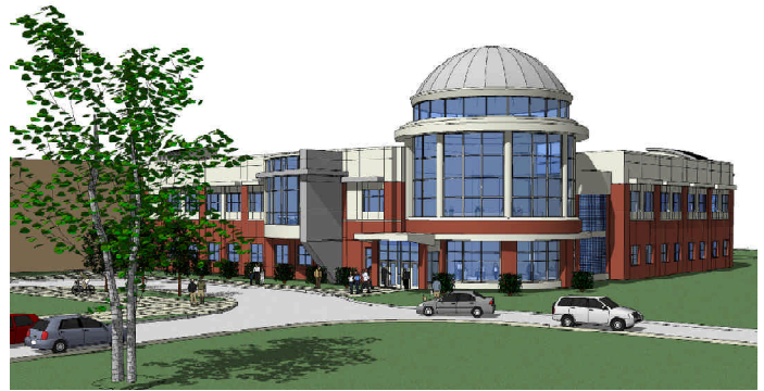
Architect's drawing of the MSU Space Science Center. Completion is expected in April 2009.
