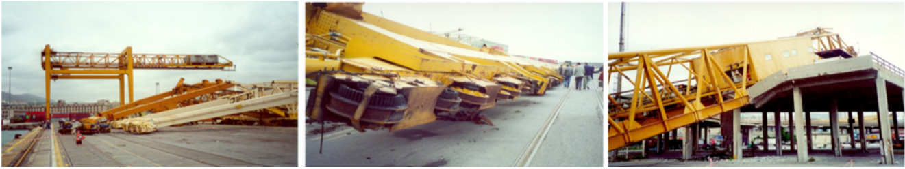
Figure 3. Damages caused by the thunderstorm downburst that occurred in the port of Genoa (Italy) on 31 August 1994 (Photos by the Authors).
