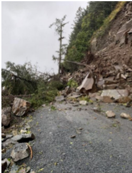
Landslide on Lowell Point Road
