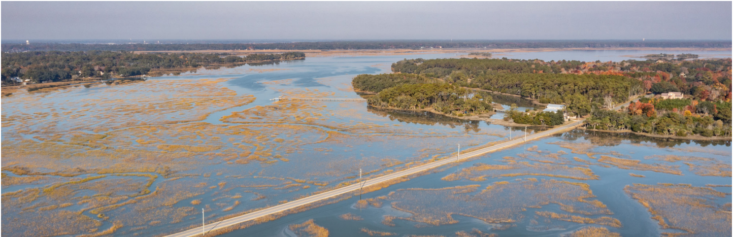
Warsaw Island causeway
