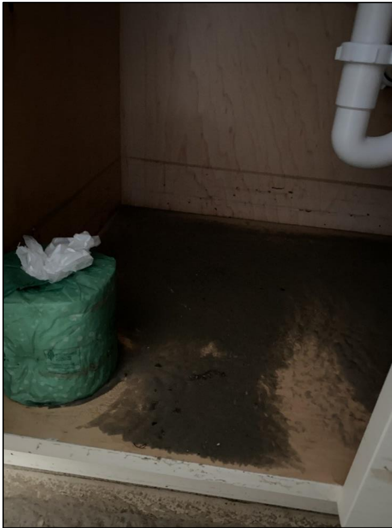
Figure 12. (a) Storm surge high water mark in bathroom cabinet on the second-story of a beachfront structure in Fort Myers Beach. (b) NWS survey team extrapolating the high water mark to the outside of the home to survey its elevation of approximately 12 ft above the brick foundation and 15 ft above MHHW. Images courtesy of the NWS.
