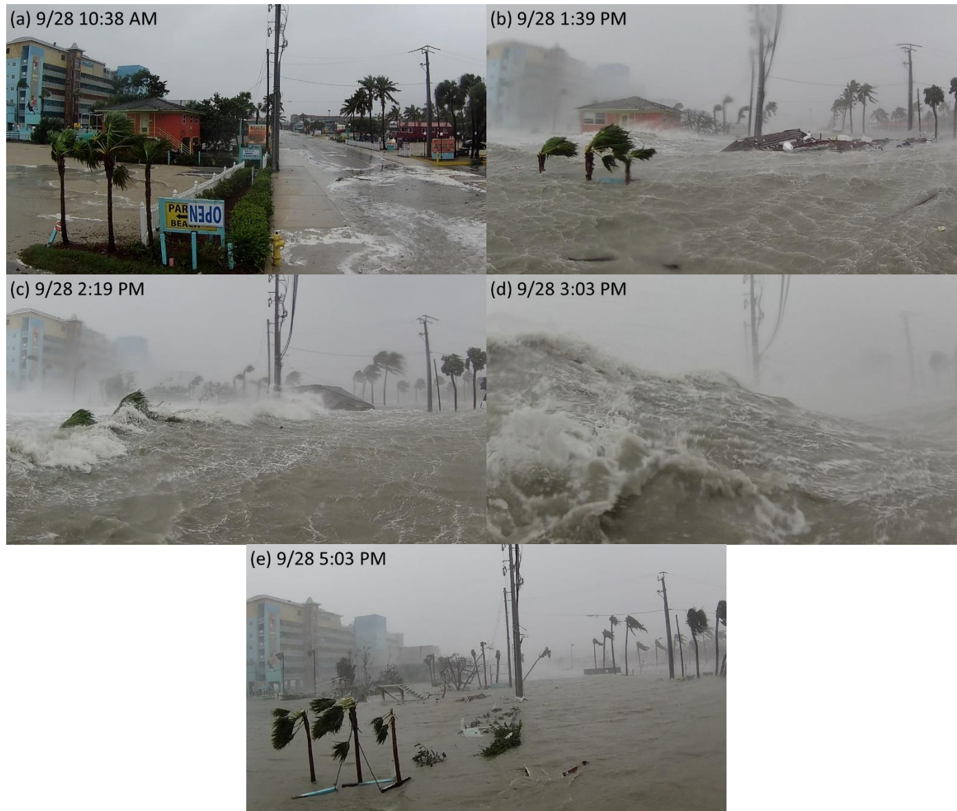
Figure 11. Series of still images and the approximate local times from a remote camera that recorded a timelapse video of storm surge inundation and destruction in Fort Myers Beach. Credit: Max Olson.
