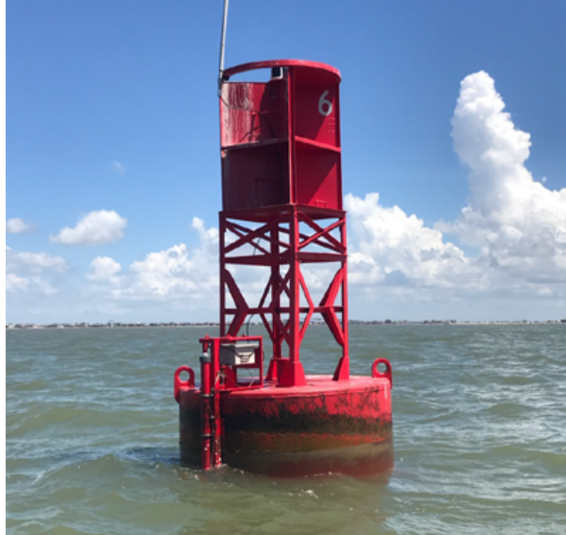
This U.S. Coast Guard Lighted Buoy 6 near the Port Freeport entrance channel in Texas has a current meter installed which feeds the Freeport, Texas Physical Oceanographic Real-time System (PORTS®) and will support navigation into and out of Port Freeport.
