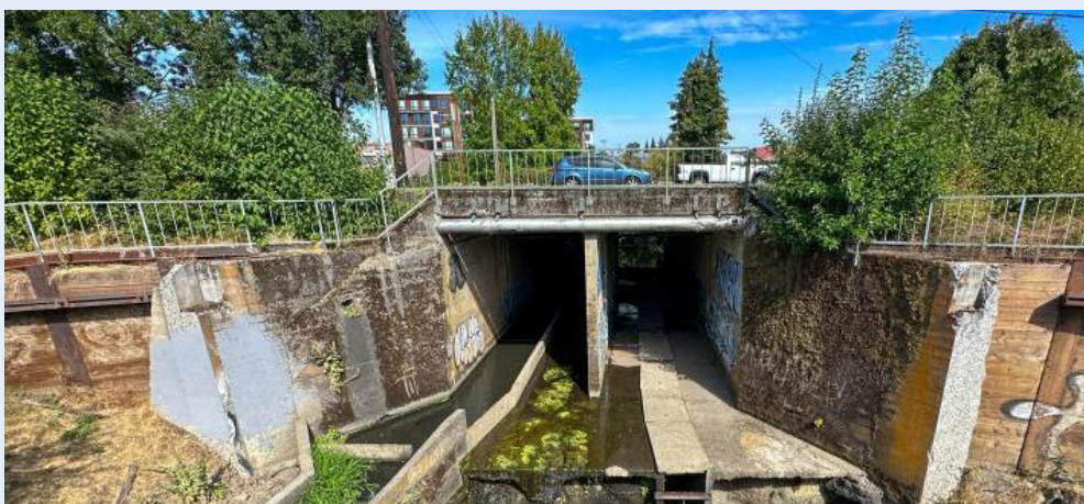
Kellogg Creek Dam. Photo credit: Jodie Robinson/NOAA.
