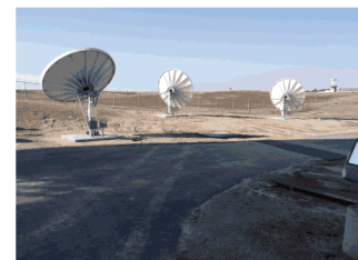
Wallops CDAS Pilot Antennas East, Spare & West
