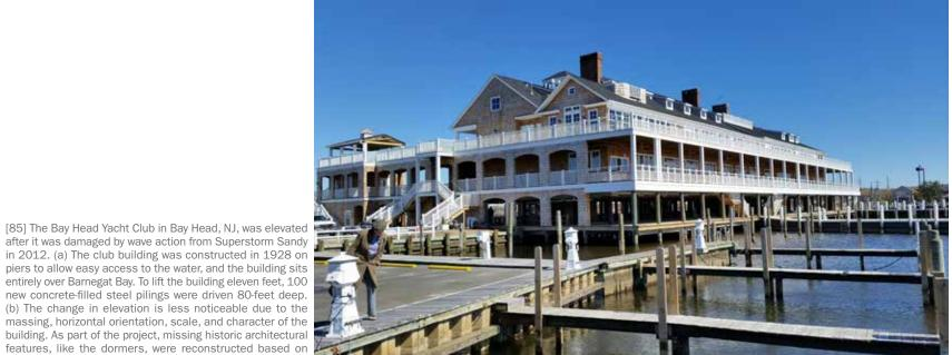
in 2012. (a) The club building was constructed in 1928 on piers to allow easy access to the water, and the building sits entirely over Barnegat Bay. To lift the building eleven feet, 100 new concrete-filled steel pilings were driven 80-feet deep. (b) The change in elevation is less noticeable due to the massing, horizontal orientation, scale, and character of the building. As part of the project, missing historic architectural features, like the dormers, were reconstructed based on
