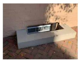
[55] A low flood wall or curb that is compatible with the historic character of the property can be constructed around basement windows to keep flood waters out. Photo: Jennifer Parker/NPS
