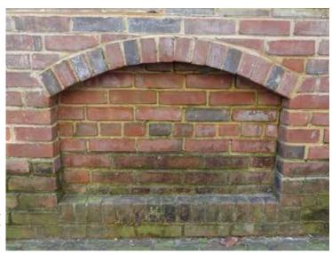
[50] To keep water out of a building, openings on secondary elevations may be permanently infilled with masonry to match or blend in with the walls. Any sills or lintels should be preserved in place, and the masonry infill should be inset to preserve the historic fenestration pattern. *Photo: Jennifer Parker/NPS*
