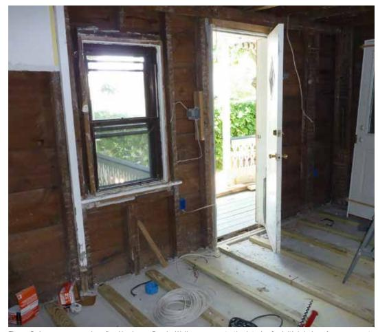
Figure 2: In-progress repairs after Hurricane Sandy. Walls are open to the interior for initial drying. A new concrete structural slab has been topped with treated wood sleepers in preparation for a new flood-damage resistant mahogany floor. Photo: Mary Delaney Krugman, JD, MSHP
