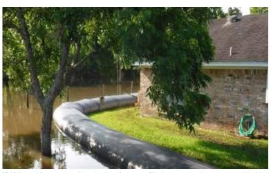
[21] A rural homeowner has deployed a water-filled temporary dam or water bladder to act as a floodwall around their residence. Water bladders require a storage area when not in use and the resources and time to fill them when a flood is imminent. *Photo: Aqua Dam, Inc*
