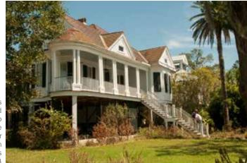
[90] While the use of architectural screening is recommended, it should generally be divided by foundation piers that have a relationship to existing porch elements. In this case, there are too few visible piers, which creates a "floating" or disconnected visual effect. Those that can be seen are undersized relative to the building and gives the impression of inadequate support. Photo: FEMA
