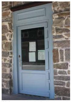
[52] Permanently installed flood barriers can be designed to be compatible with a building's historic features and character, as with this operable flood door on a circa 1770 commercial building in Ellicott City, MD. *Photo: Liz Petrella/NPS*
