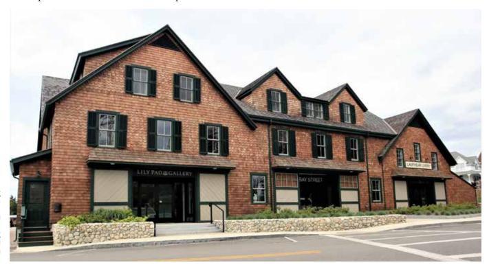
Figure 5: View of the building after the floodproofing and rehabilitation project was complete. The historic barn doors and many historic windows were preserved. Damaged or missing shingle siding was replaced in kind. The foundation is now two feet taller than it was at the start of the project. Wet floodproofing of the first floor provides additional resiliency and protection for floods that exceed the new elevation height. *Photo: Pariseault Builders*
