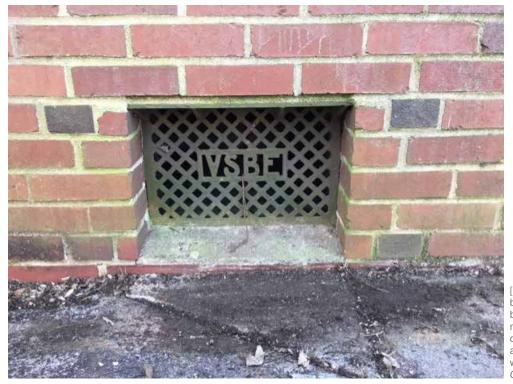
[56] To create a watertight seal around the building, any existing vents or openings below the established flood risk level must be sealed during a flood. Vents that cannot be sealed internally will require an exterior and/or interior cover to keep water from entering the building. *Photo: Chelius Carter*
