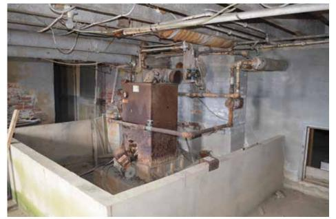
[42] Mechanical equipment that remains in a basement that is likely to flood should be enclosed behind waterproof walls. The walls may be partial height, as shown in this example, if flood waters are not expected to exceed that height. In other cases, waterproof enclosures must fully surround the equipment, which can be accessed by submarine-quality doors or hatches. *Photo: Quinn Evans*
