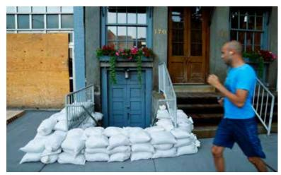
[20] Temporary measures such as sandbags can be a simple and inexpensive solution for protecting buildings in low-lying and vulnerable areas, but they are not meant to withstand moving floodwaters for extended time periods. *Photo: Eduardo Munoz/Reuters*
