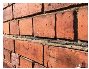
[66] In order to limit the absorption of flood waters, a horizontal waterstop joint can be installed in a building's walls depending upon the wall material and construction. This was also done historically, as shown in this historic brick wall with slate embedded in the mortar to limit water wicking up the wall. *Photo: eagle/stock.adobe.com*
