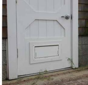
[63] When new venting is required, the placement and design should be compatible with the existing property. The insulated, engineered vent added to the door of this property in Sandy Hook, NJ, has been painted to blend in. *Photo: Tina Roach*
