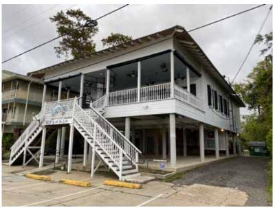
[89] This building in Louisiana has been raised on piers, but the foundation piers are set back from the face of the building, do not line up with the porch posts, and are visually undersized. New foundation piers, posts, and columns should have a visual appearance that more closely matches traditional foundation placement, size, and materials, even if that requires wrapping more modern, slender steel members with a masonry veneer. *Photo: Roderick Scott*
