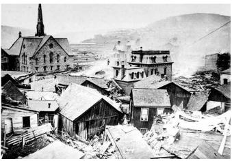
[10] The Great Johnstown Flood of 1889, caused by a catastrophic dam failure, shows the extent of damage that can occur from a large-scale, fast-moving flood event. Whole buildings were destroyed, others were shifted from their foundations, and massive amounts of debris caused considerable loss of life, damage, and destruction. *Photo: NPS*
