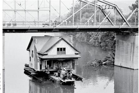
[109] At times, moving a house over water may provide more space to maneuver and facilitate keeping the building in one piece as it is moved. Photo: Courtesy of mywvhome.com
