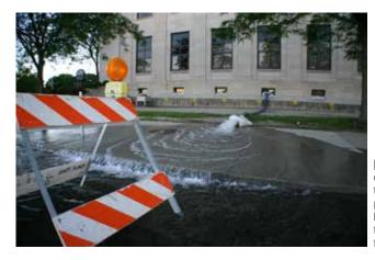
[65] Flood waters often must be actively pumped out of and away from the property, as seen in this image from Des Moines, IA. The pumping process should be designed to control the shift in hydrostatic pressure on the building and remove all flood waters that do not naturally drain or recede from the property. *Photo: Chris Snider*
