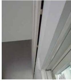
Figure 4: Crown molding covers an opening at the top of walls to allow air to circulate and dry wall cavities after a flood, seen here before the sacrificial insulating foam strip has been applied. *Photo: Mary Delaney Krugman, JD, MSHP*
