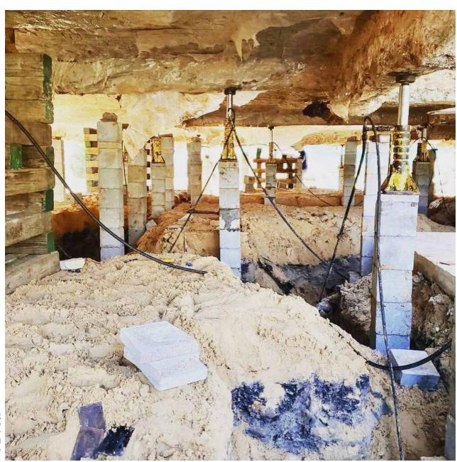
[79] Buildings on a concrete slab can be more challenging to lift. In some cases, as shown in this example, the existing slab can be lifted and still remain the floor for the interior spaces. In other instances, the slab may need to remain at grade, with a new elevated floor structure constructed above. *Photo: p3elevation.com*
