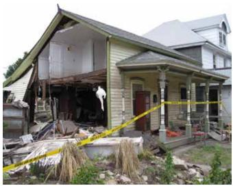
[8] Understanding the characteristics of a flood are critical to understanding property risk. Significant structural damage occurred to this building as a result of a riverine flood in Cedar Rapids, IA, in 2008. *Photo: Greg Januska*
