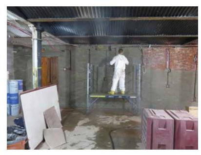
[48] A waterproof coating is applied to the interior surface of lower-level walls of the public library in Hoboken, NJ. Prior to applying such a coating, the product should be researched by building science professionals with knowledge of historic materials and methods to ensure that the coating will not cause damage to or accelerate deterioration of the structure. Photo: David V. Abramson for Hoboken Public Library
