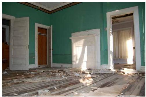
[59] Flood waters can have a significant impact on historic building interiors. Historic features and materials can often be retained and repaired and should not be preemptively removed or replaced. Much of the interior of this flooded historic property in Gulfport, MS, was able to be cleaned and retained. *Photo: Jenifer Eggleston/NPS*
