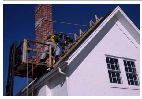
[113] Fragile features like chimneys should be evaluated and braced before a building is moved. *Photo: Mike Booher/NPS*
