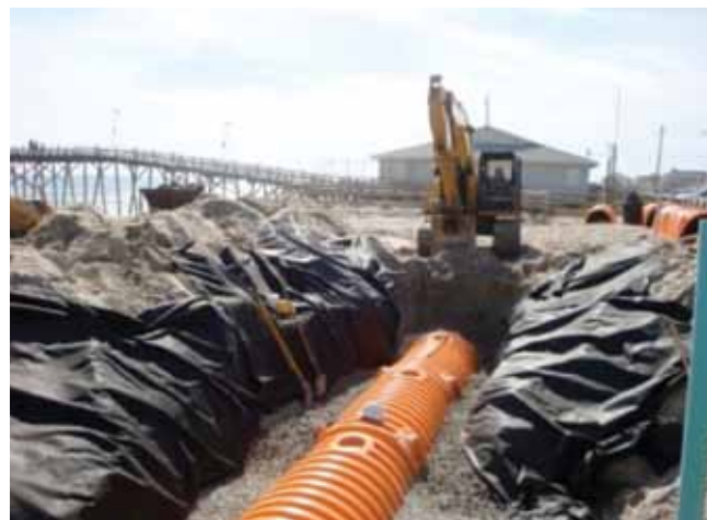
Dune filtration unit under construction at Kure Beach.
