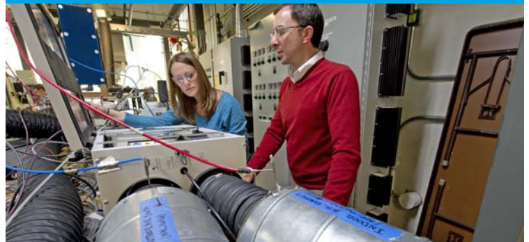
Researchers accurately monitor the nation's emerging efficiency products for indoor comfort at the Advanced HVAC Systems Laboratory. Photo by Dennis Schroeder, NREL/PIX 20008
