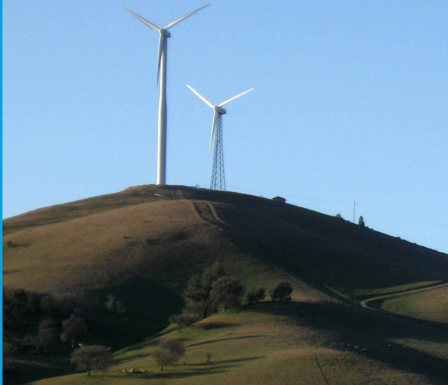
Tehachapi Pass Wind Farm in California. The 705-megawatt farm is composed of about 5,000 wind turbines. Photo by David Hicks, NREL 18459
