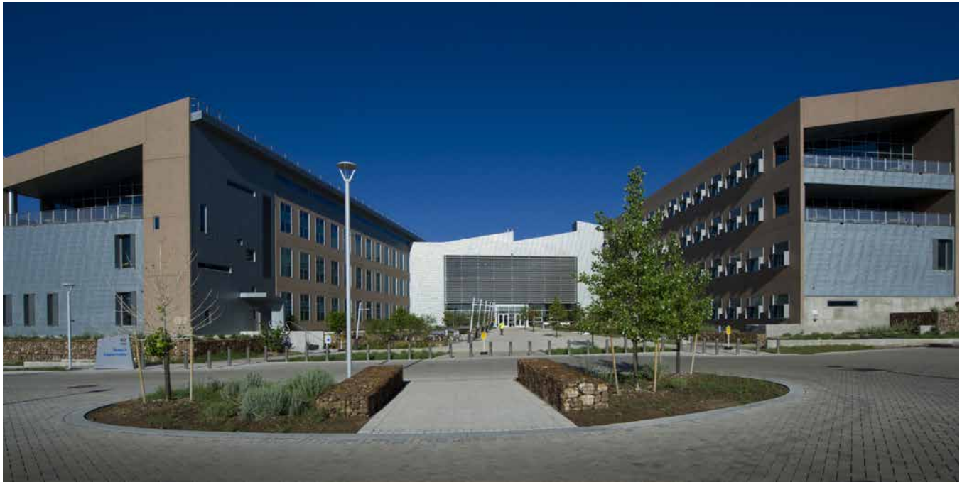
Front view of the Leadership in Energy and Environmental Design (LEED) Platinum certified Research Support Facility. Photo by Dennis Schroeder, NREL 19350
