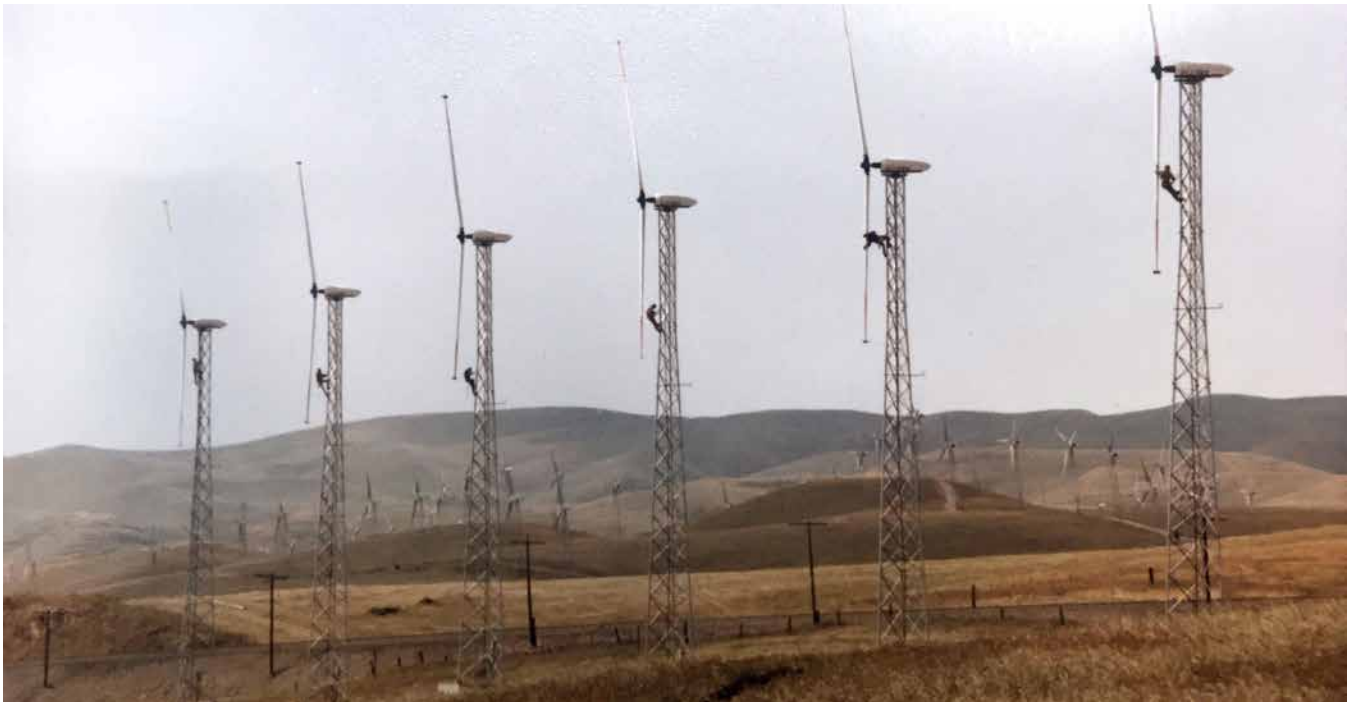
Blade washing crews working on ESI-54 wind turbines on Jess Ranch in Altamont Pass, California in 1985. Photo by Walt Musial, NREL
