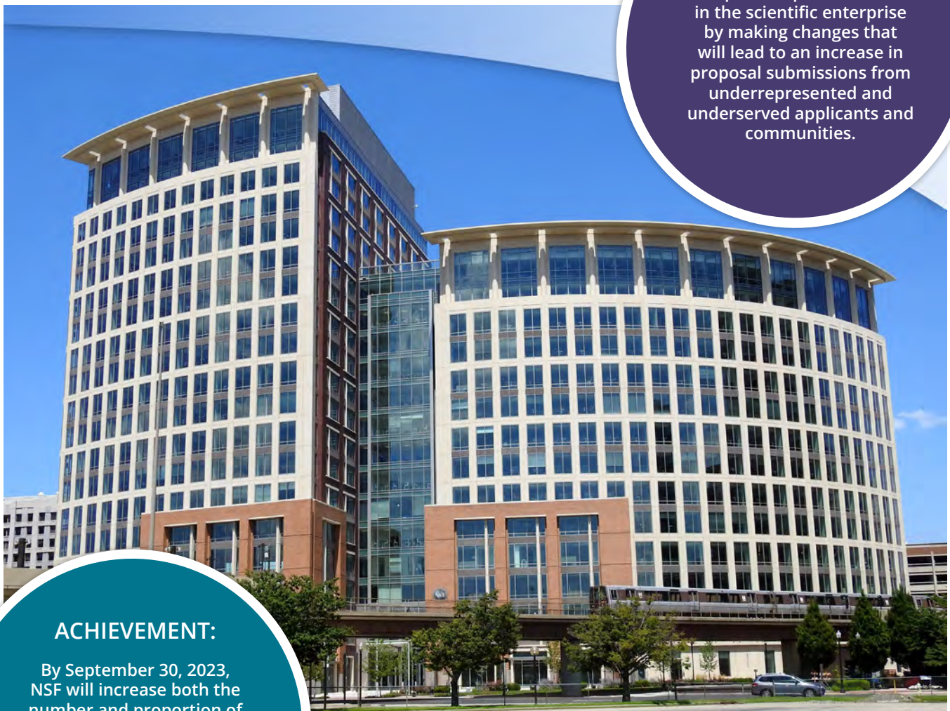
NSF Headquarters in Alexandria, VA.: Credit: NSF
