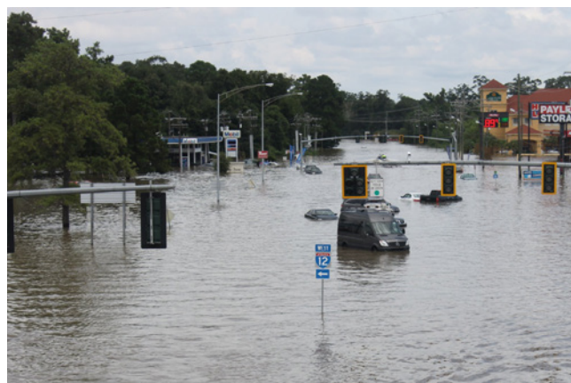
Flooded businesses in Baton Rouge, LA, August, 2016.
