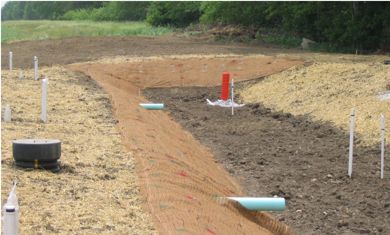
Treatment Wetland under Construction
