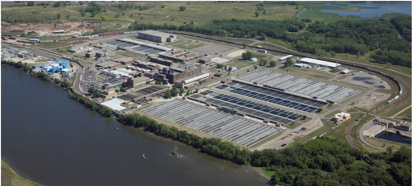
Metropolitan Wastewater Treatment Plant
