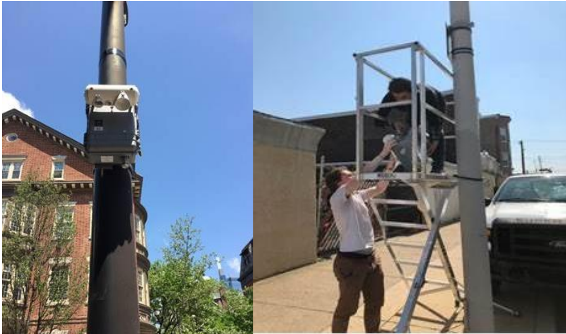
Figure 2. Sampling unit mounted on a street pole
